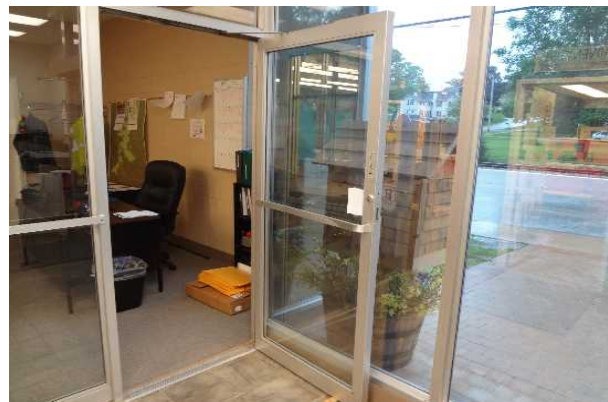
#34: INTERIOR DOOR, FULLY-GLAZED ALUMINUM-FRAMED SWINGING
