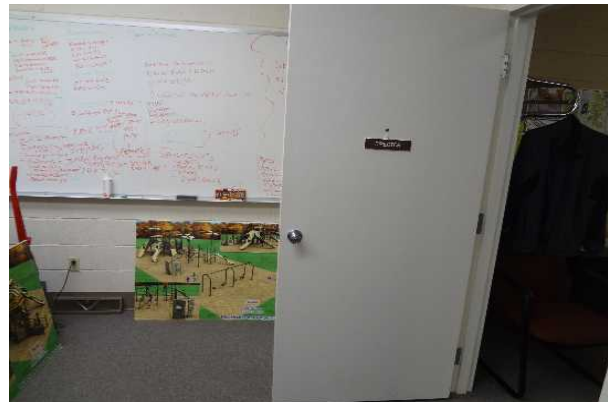
#32: INTERIOR DOOR, WOOD HOLLOW-CORE
