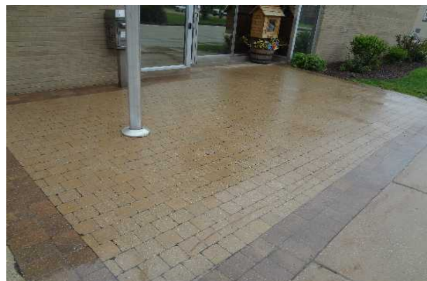
#6: SIDEWALK, CLAY BRICK/MASONRY PAVERS
