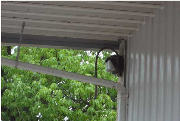
#25: HIGH PRESSURE SODIUM LIGHTING FIXTURE
