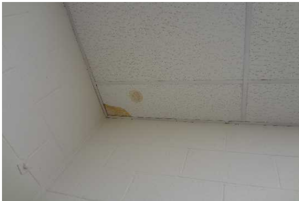
#39: STAINED ACOUSTICAL CEILING TILE
