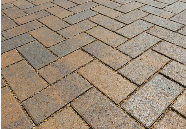
Figure 70 - Pervious Pavers (Techniseal)
