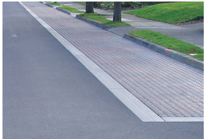
Figure 39 - Permeable Parking Pavers (Village of Shorewood)
