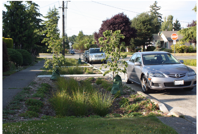
Figure 51 - Roadside Swale (Green Infrastructure Digest)
