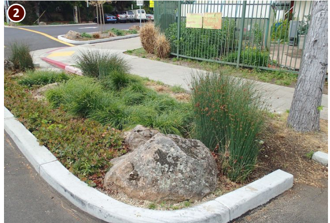
Figure 40 - Stormwater Bulb-Out (Toni Best)
