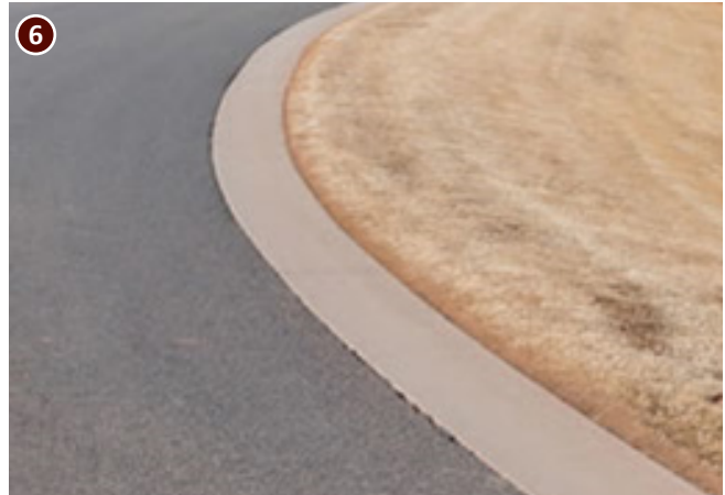
Figure 54 - Rolled Concrete Apron (Specify Concrete)
