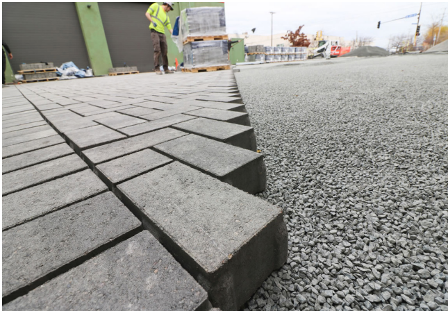
Figure 71 - Pervious Pavers (MWMO)
