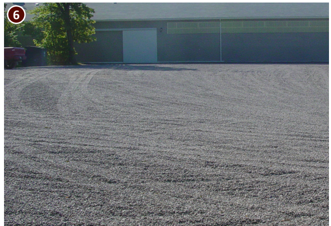
Figure 20 - Well Maintained Gravel Surface (Dare Inc.)
