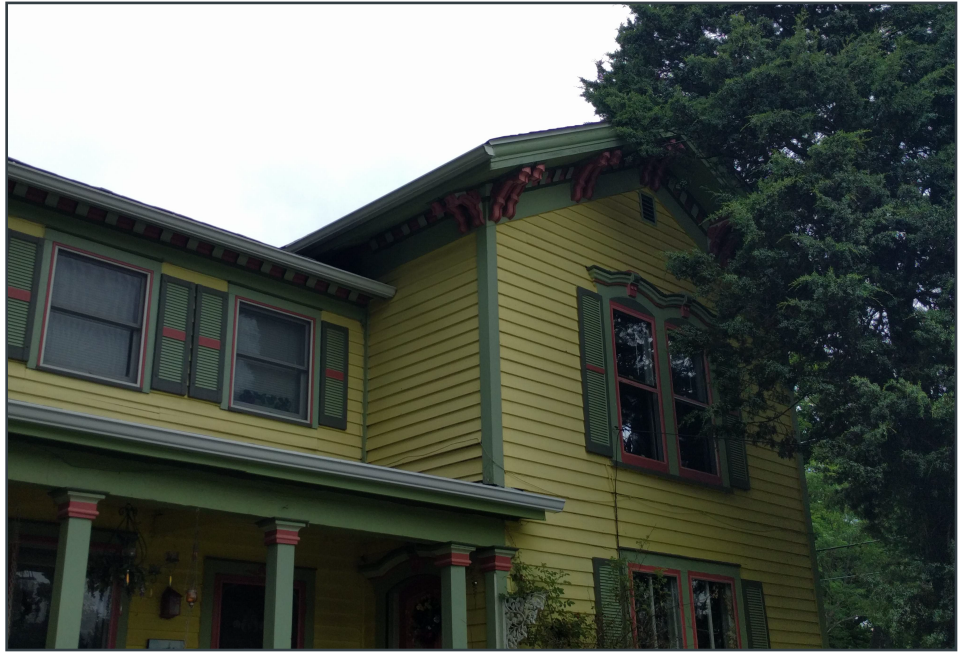
Image 22: Covering up wood siding can obscure or erase completely architectural elements that help make your home unique.
