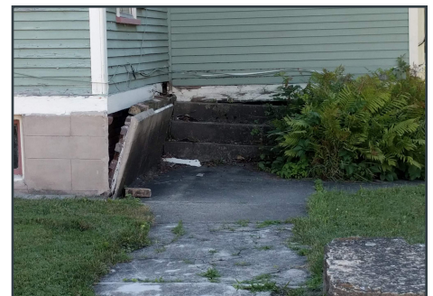
Image 6: Dangerous Settling around the Foundation
