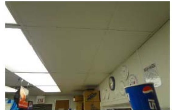
#33: INTERIOR CEILING FINISH, ACOUSTICAL TILE (ACT)
