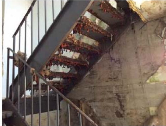
PHOTO #37: SOUTH STAIRS
