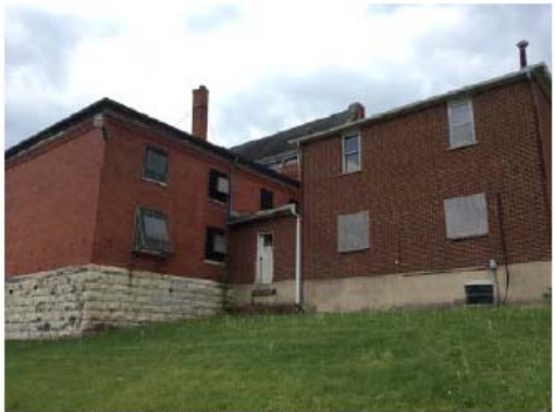
PHOTO #3: NORTH ELEVATION
