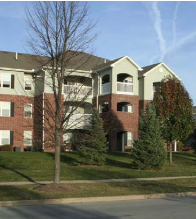
Fox River Subdivision Multifamily Residential
