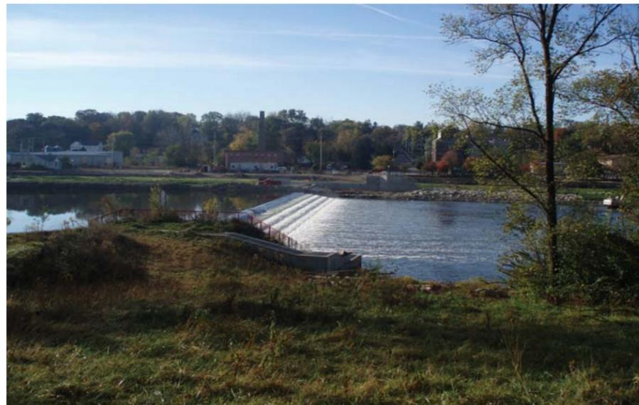
Construction of a denil fish ladder adjacent to the dam's north abutment allows to pass fish and to provide water supply to the north shore of the river during low flow conditions.
