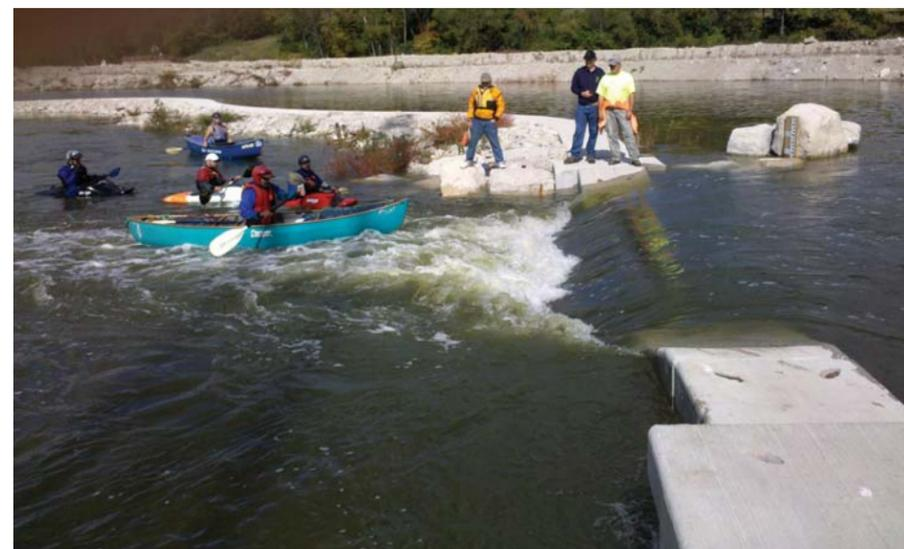
Partial dam removal allowed the construction of an 1100 foot long fish/canoe bypass channel and divider island along the south shore of the river. An access bridge to the divider island is scheduled to be constructed in 2011, and a new stream gage has been installed.
