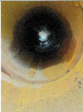
Interior pipe in good condition, no signs of erosion/corrosion, typ.
