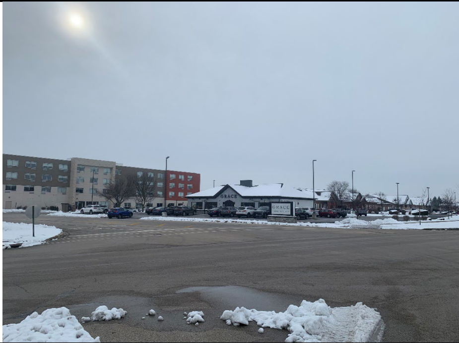
COUNTRYSIDE PARKWAY – WESTBOUND APPROACH
