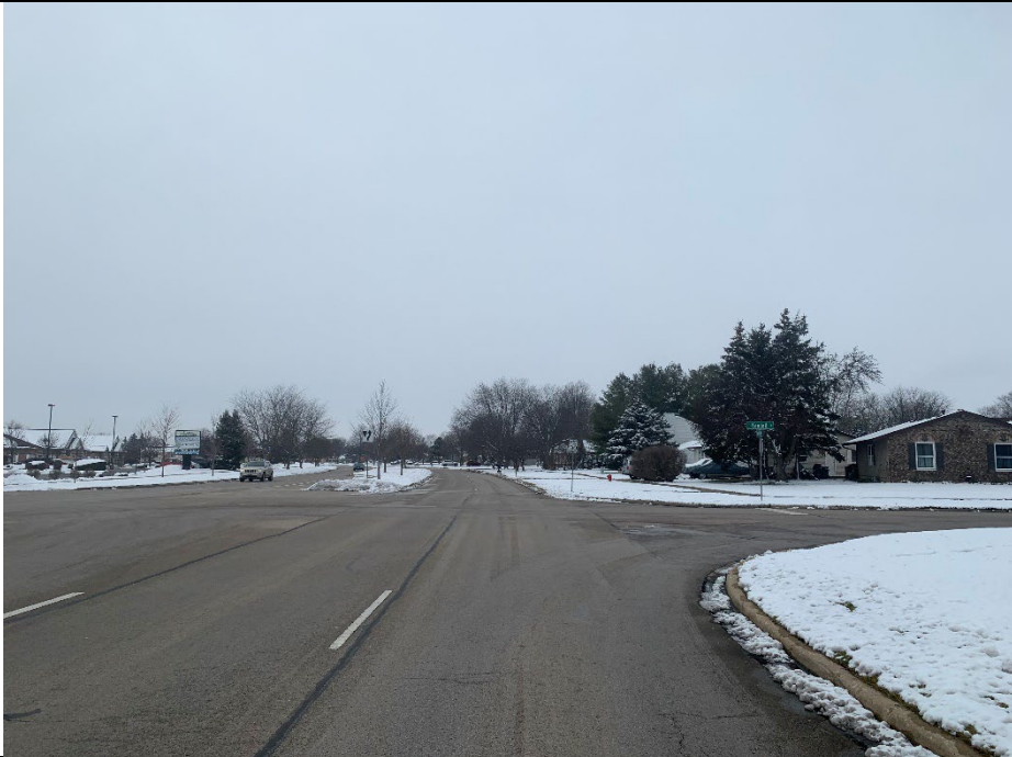
COUNTRYSIDE PARKWAY – WESTBOUND APPROACH
