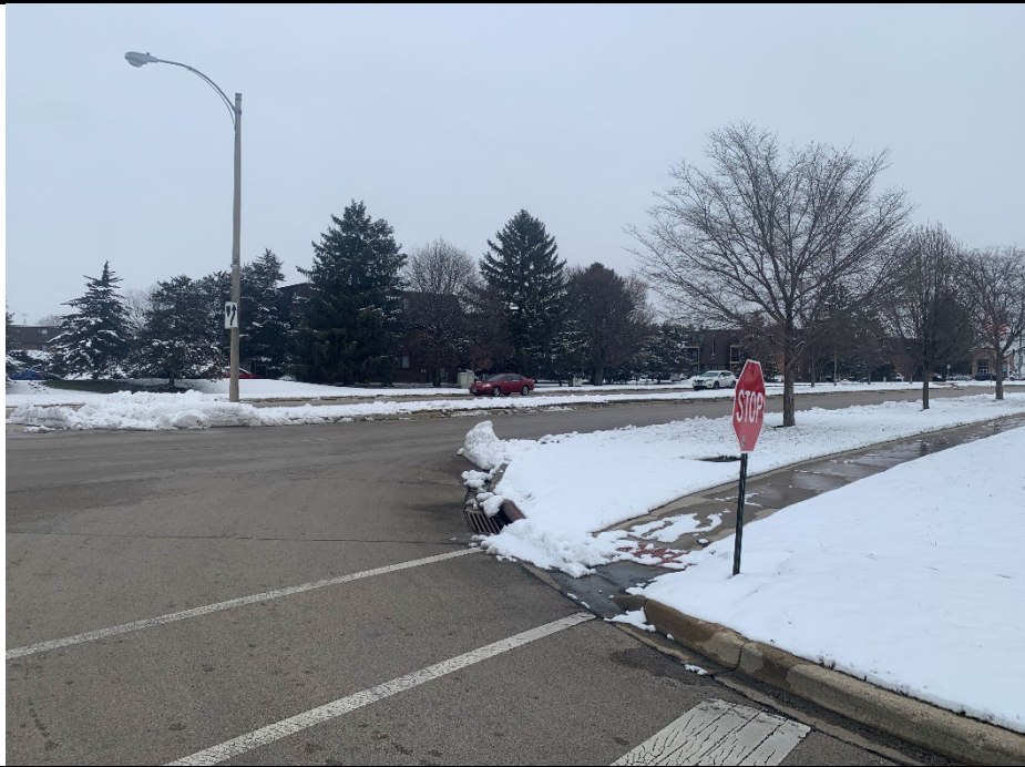
EAST KENDALL DRIVE – NORTHBOUND APPROACH LOOKING EAST
