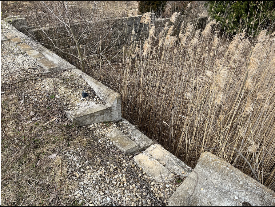
MISSING RETAINING WALL BLOCKS
