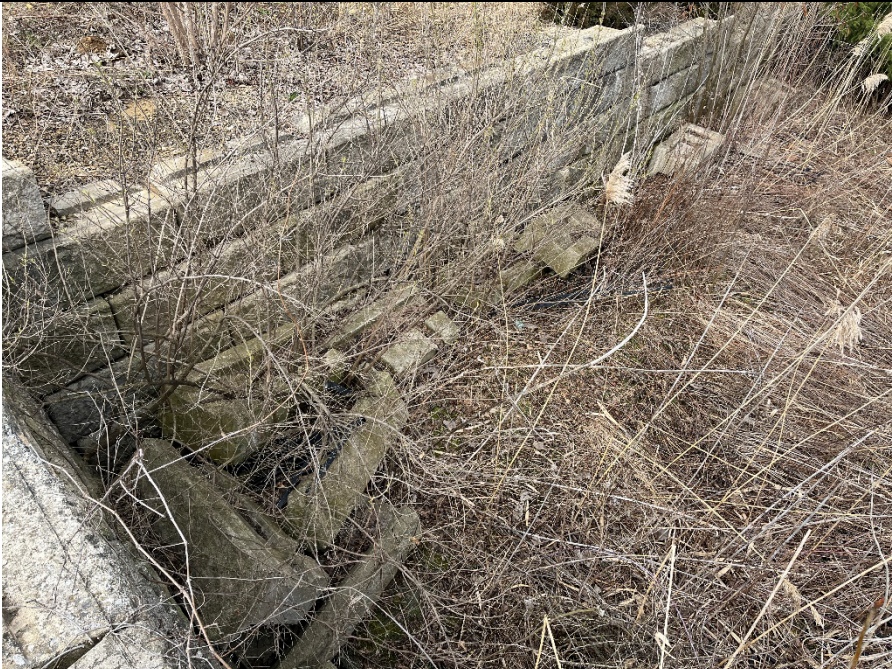
FALLEN RETAINING WALL BLOCKS
