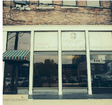
Rear Facade Example.
