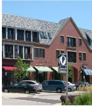
Primary Materials: Brick
