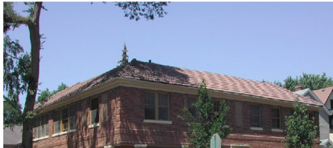
Roof Materials: Ceramic Tile
