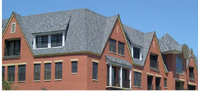
Roof Materials: Asphalt Composite Shingles
