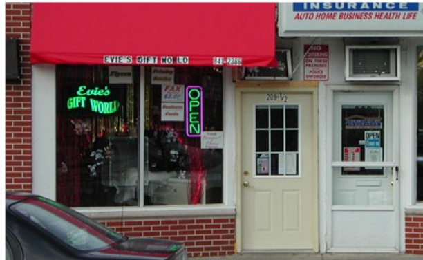
Prohibited: Residential Grade Doors on Commercial Buildings.
