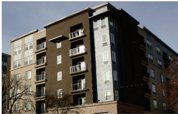
Figure 10-21-4K (8). Balconies Integral to Facade.
