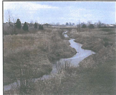
Drainage swale utilizes natural drainage patterns
