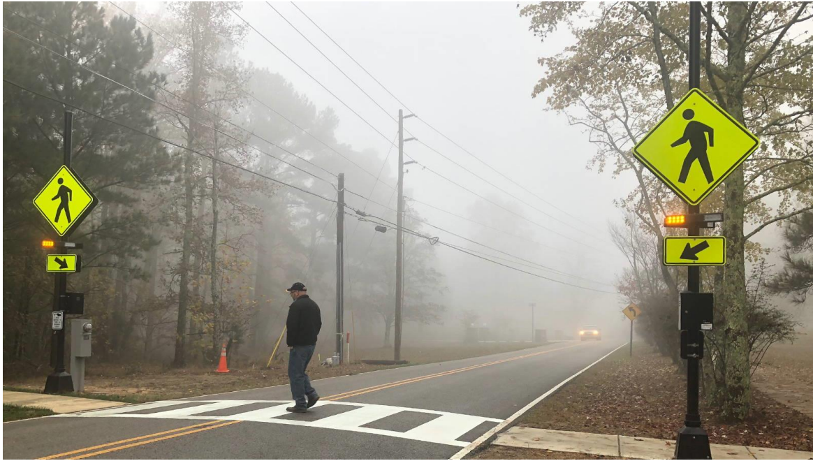
Photo 3. Sample RRFB Installation (TAPCO)
