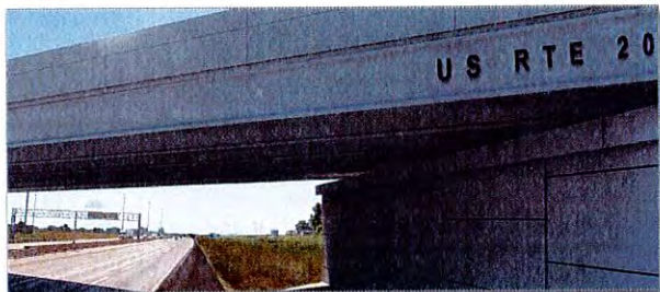
Proposal Alternative - MSE Wall Abutment
