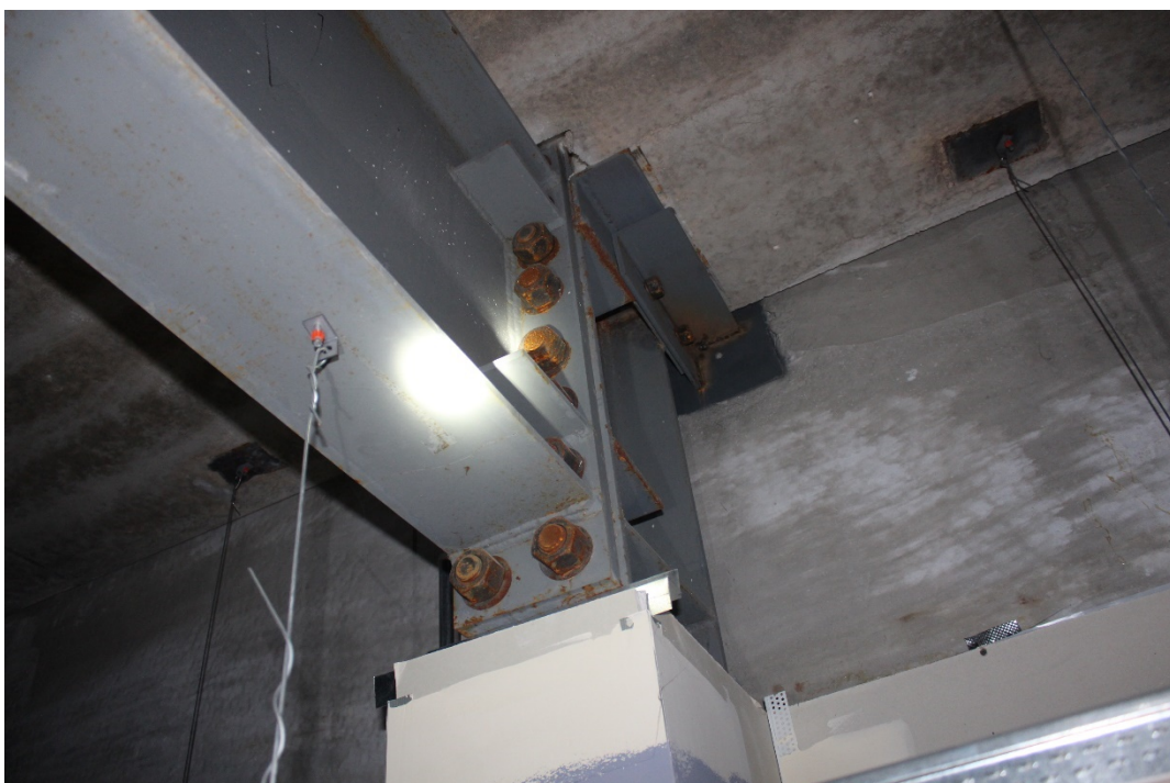
Photograph 4 – Moment Connection in Steel Frame (Consistent w/ Existing Building Drawings)
