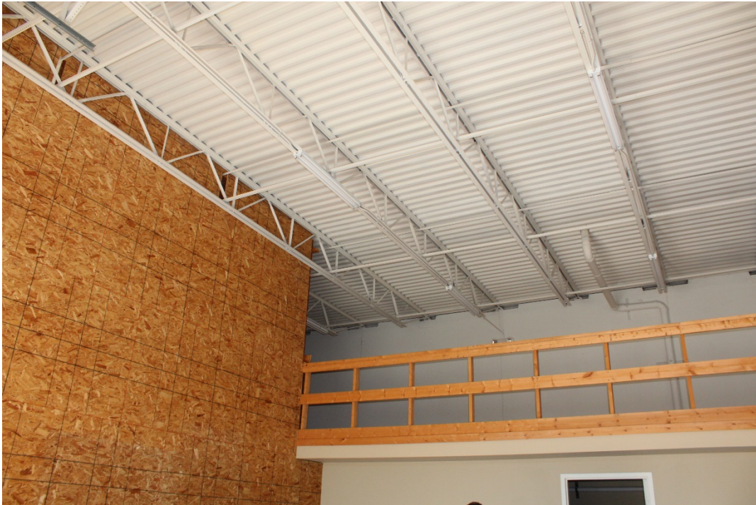
Photograph 7 – Steel Roof Framing of Shed (Consistent w/ Existing Building Drawings)
