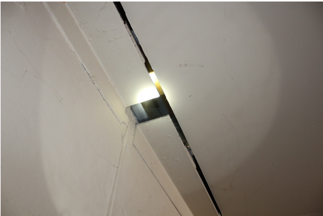
Photograph 8 – Partially Visible Light-Gage Steel Mezzanine Floor Framing (Consistent with Existing Building Drawings)
