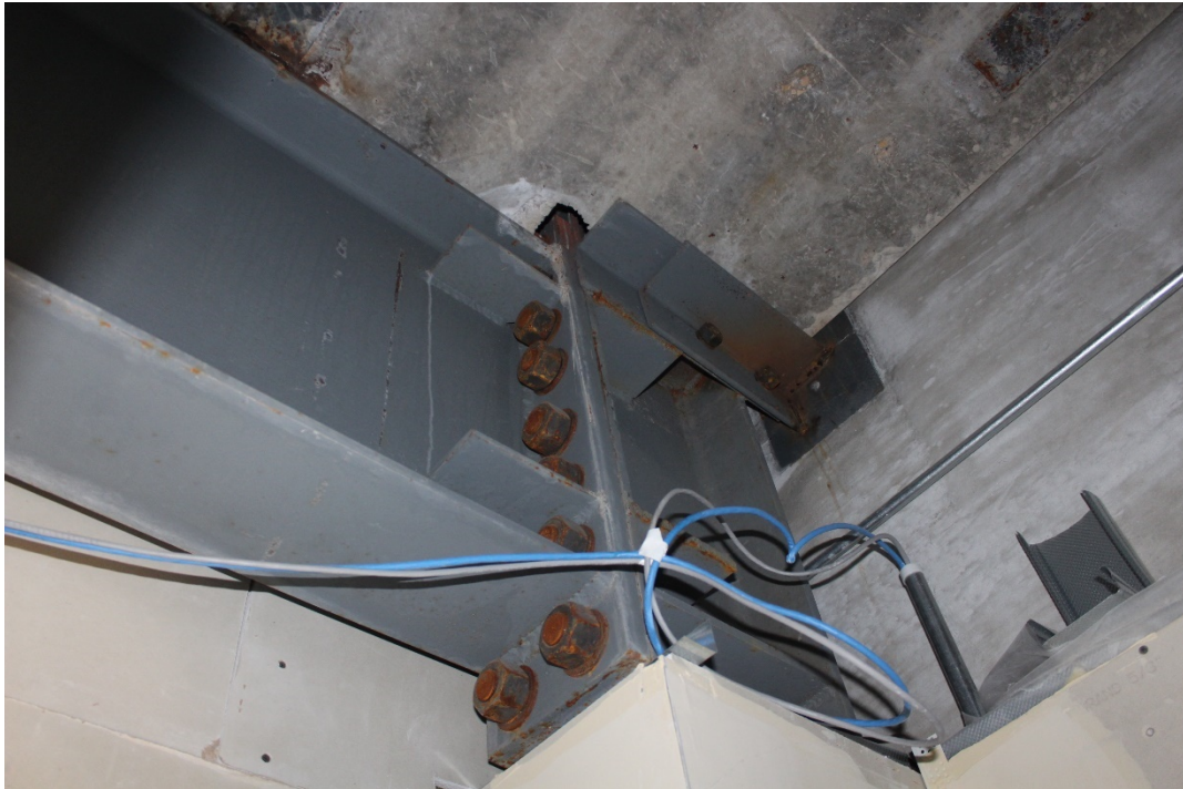
Photograph 6 – Moment Connection in Steel Frame (Consistent w/ Existing Building Drawings)
