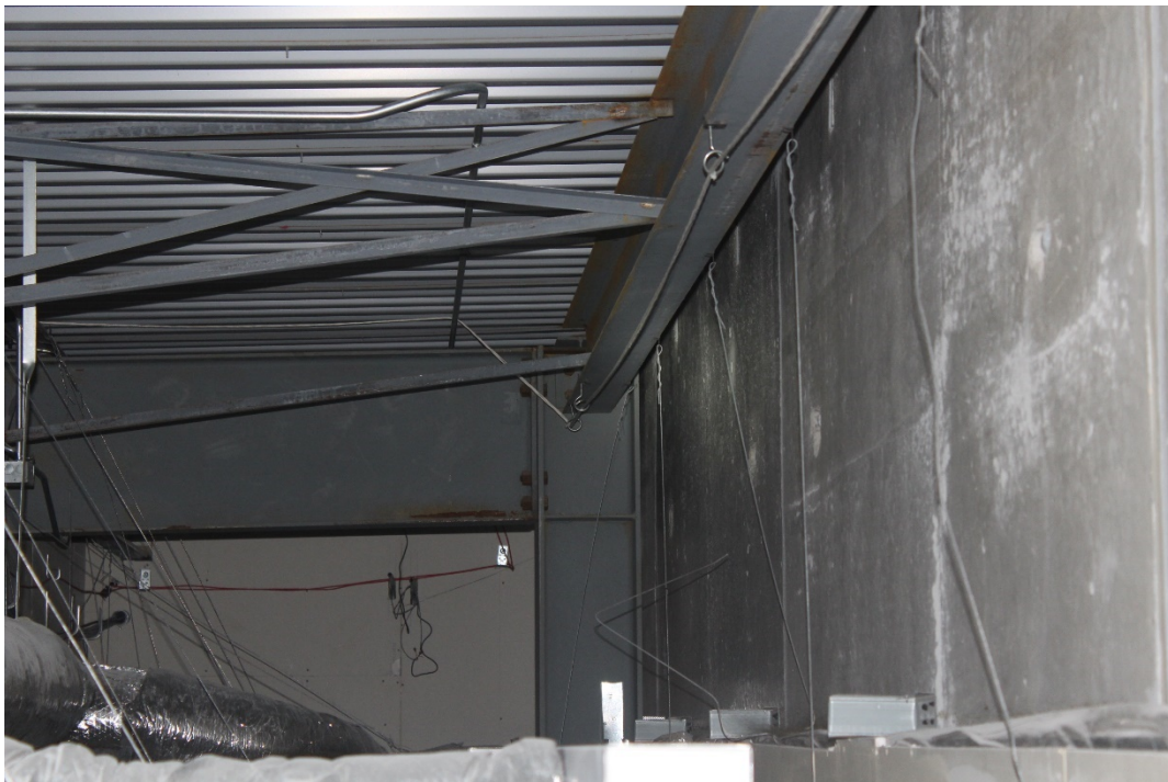
Photograph 6 – Moment Connection in Steel Frame (Consistent w/ Existing Building Drawings)
