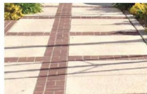
Figure 15 - Improved Sidewalk Pavement (California DOT)
