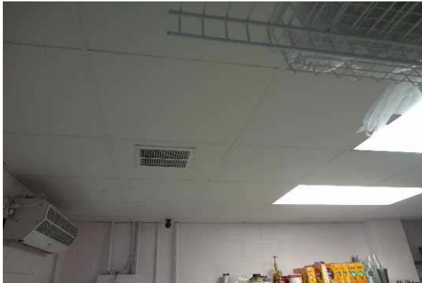
#49: INTERIOR CEILING FINISH, ACOUSTICAL TILE (ACT) - FOXY'S ICE CREAM
