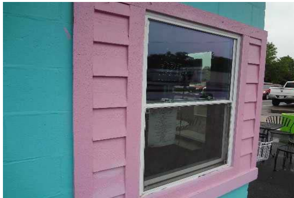
#13: WINDOW, VINYL-CLAD DOUBLE-GLAZED 12 SF
