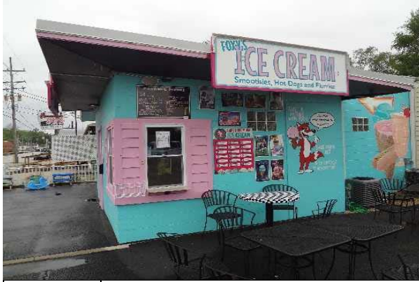
#11: EXTERIOR WALL, PAINTED SURFACE
