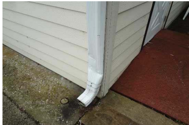
#10: DAMAGED DOWNSPOUT
