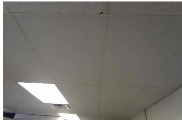
#48: INTERIOR CEILING FINISH, (ACT) DROPPED FIBERGLASS - GINGER + SOUL
