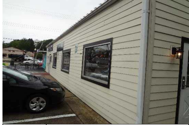
#12: EXTERIOR WALL, VINYL SIDING
