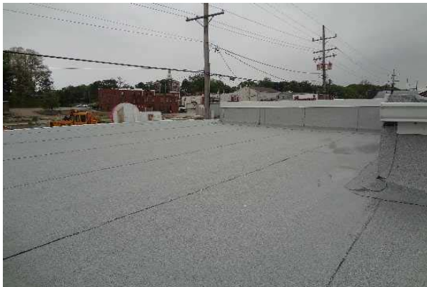
#9: ROOF, MODIFIED BITUMINOUS
