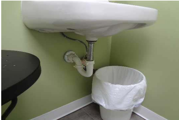
#7: ADA, RESTROOM, LAVATORY PIPE WRAPS
