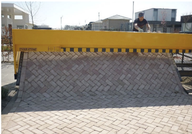
Figure 72 - Paver Laying Machine (Detroit News)
