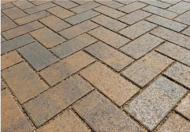
Figure 70 - Pervious Pavers (Techniseal)
