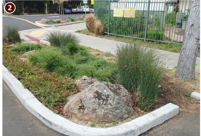
Figure 40 - Stormwater Bulb-Out (Toni Best)
