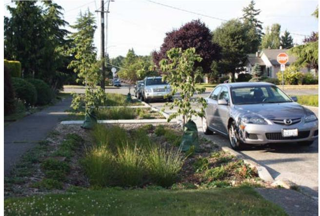
Figure 51 - Roadside Swale (Green Infrastructure Digest)
