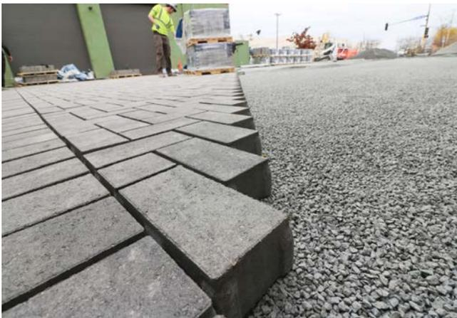
Figure 71 - Pervious Pavers (MWMO)
