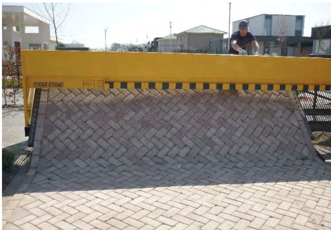
Figure 72 - Paver Laying Machine (Detroit News)
