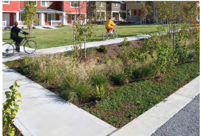
Figure 52 - Roadside Swale (Mithun)
