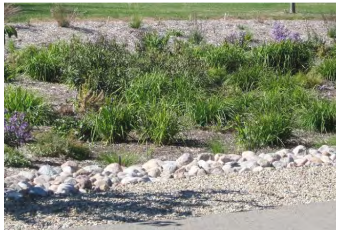
Figure 68 - Rain Garden Off Curbless Street (Prairie Rivers)
