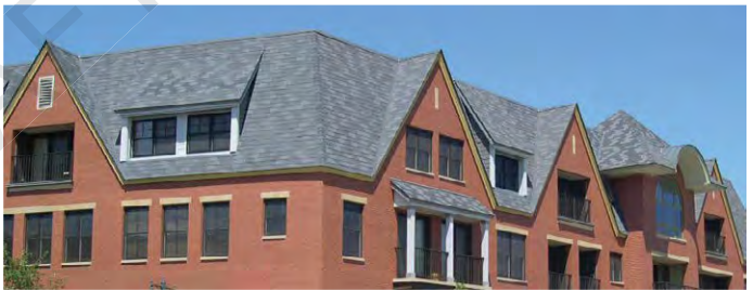
Roof Materials: Asphalt Composite Shingles
