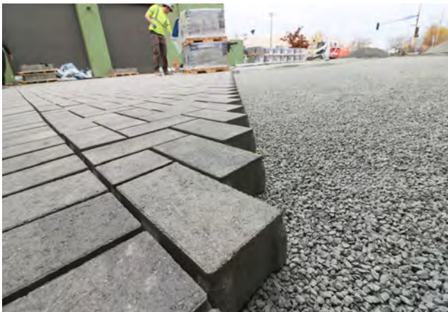
Figure 71 - Pervious Pavers (MWMO)
