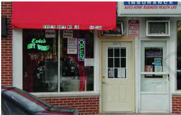
Prohibited: Residential Grade Doors on Commercial Buildings.
