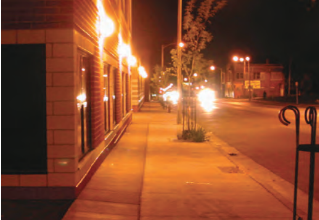
Figure 64 - Street Lighting “Don’t” (Farr Associates)
