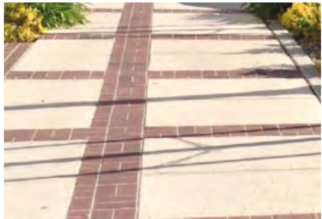
Figure 15 - Improved Sidewalk Pavement (California DOT)
