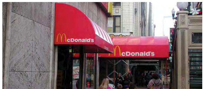
Prohibited Awnings: Canopy awnings that extend from the front facade into the right-of-way
