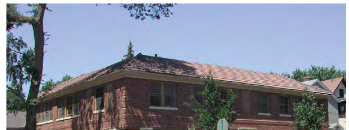
Roof Materials: Ceramic Tile
