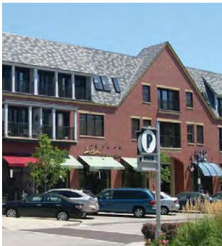
Primary Materials: Brick
