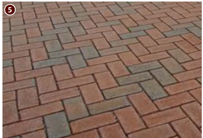
Figure 42 - Permeable Pavers (Terran Capital)
