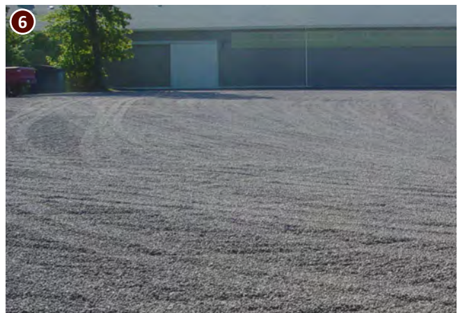
Figure 20 - Well Maintained Gravel Surface (Dare Inc.)
