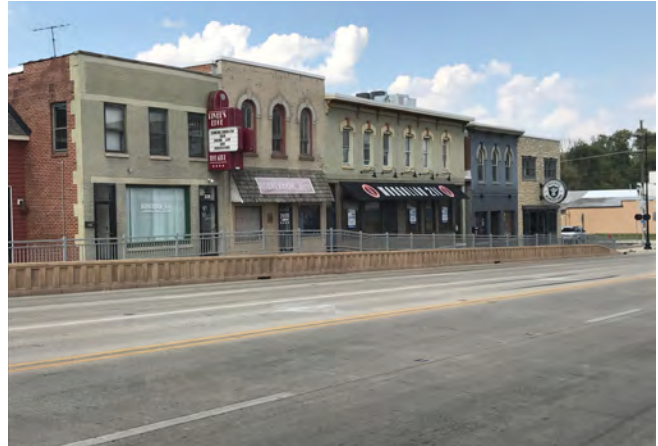
Figure 6 - Bridge Street Facades (Farr Associates)
