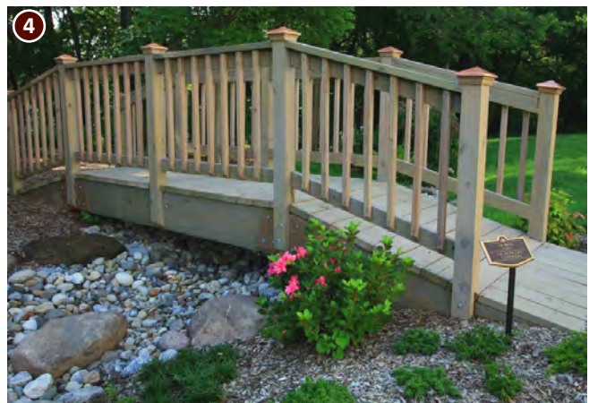
Figure 56 - Bridge Over Swale (Chesapeake Dock)
