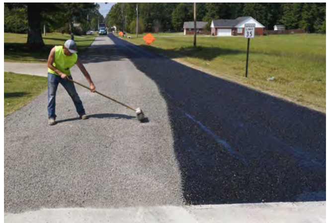
Figure 48 - Road Resurfacing (Decatur Daily)
