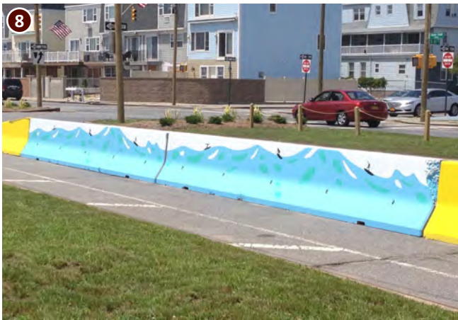
Figure 11 - Painted Concrete Barrier (NYC Parks)
