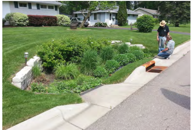
Figure 67 - Residential Rain Garden (Metro Blooms)
