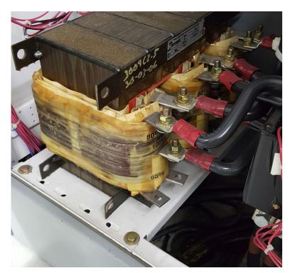
Image 1: This is a picture of the autotransformer that needs replacing.
