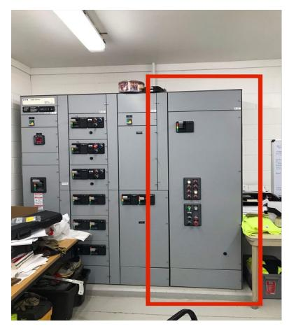
Image 2: This is a picture of the motor control cabinet for Well 4 where the autotransformer is housed.
