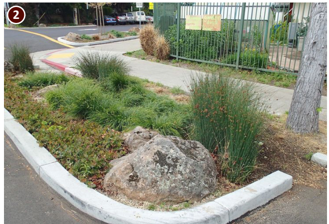
Figure 40 - Stormwater Bulb-Out (Toni Best)
