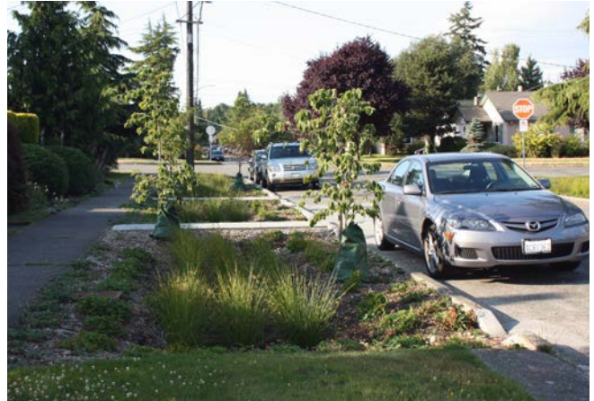
Figure 51 - Roadside Swale (Green Infrastructure Digest)
