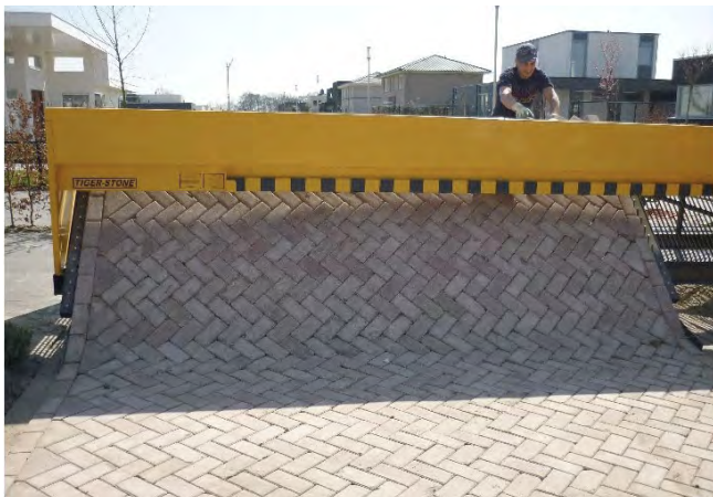
Figure 72 - Paver Laying Machine (Detroit News)
