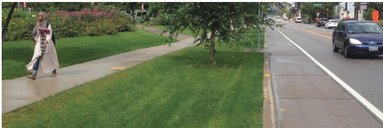
Figure 50 - Basic Roadside Swale (NACTO)
