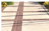
Figure 15 - Improved Sidewalk Pavement (California DOT)
