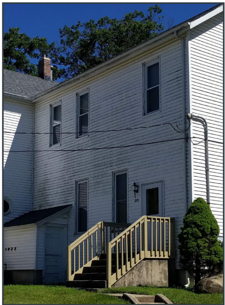
Image 5: Mold & Mildew prefer places that are damp such as basements, crawlspaces, foundations, as well as on building faces that receive minimal sun (Above)
