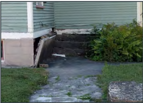
Image 6: Dangerous Settling around the Foundation
