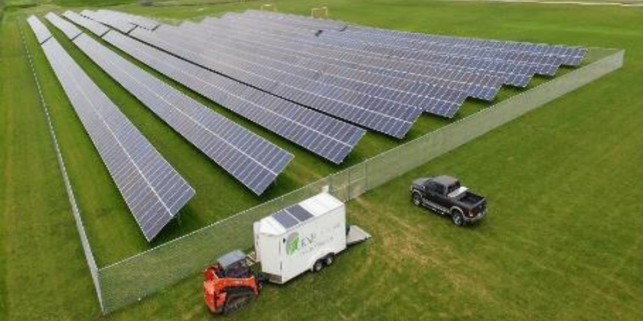
Tri-Creek School Corporation, Lowell Indiana 1MW SOLAR ARRAY 3,936 SOLAR MODULES 728 TONS OF CO2 REDUCED PER YEAR
