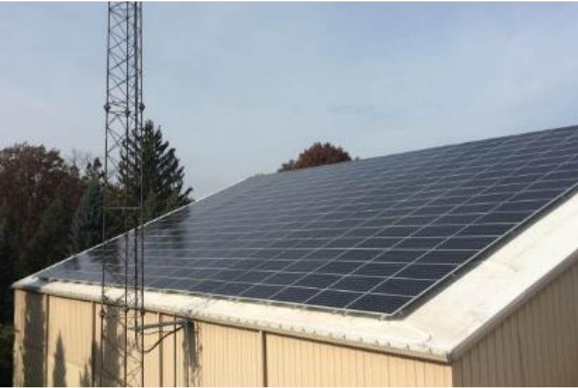
The Summit, Ft. Wayne, Indiana 100 kW SOLAR ARRAY 323 SOLAR MODULES 73 TONS OF CO2 REDUCED PER YEAR
