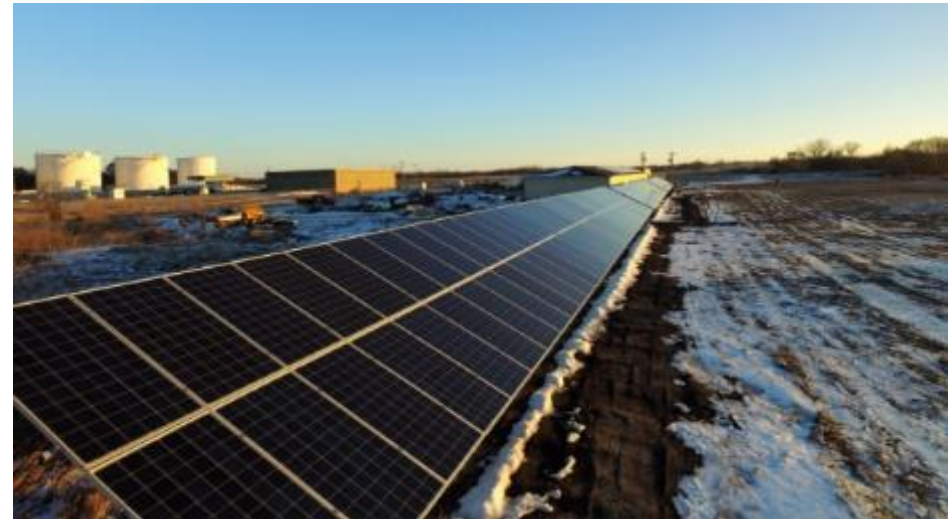
JAX Properties 100 kW SOLAR ARRAY 327 SOLAR MODULES 73 TONS OF CO2 REDUCED PER YEAR
