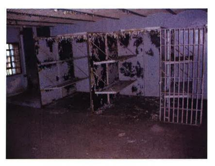
7. View of peeling Lead-Based Paint in the basement.
