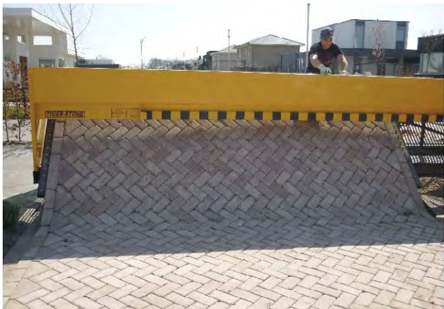
Figure X - Paver Laying Machine (Source)
