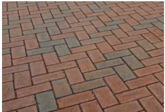
Figure X - Permeable Pavers (Source)
