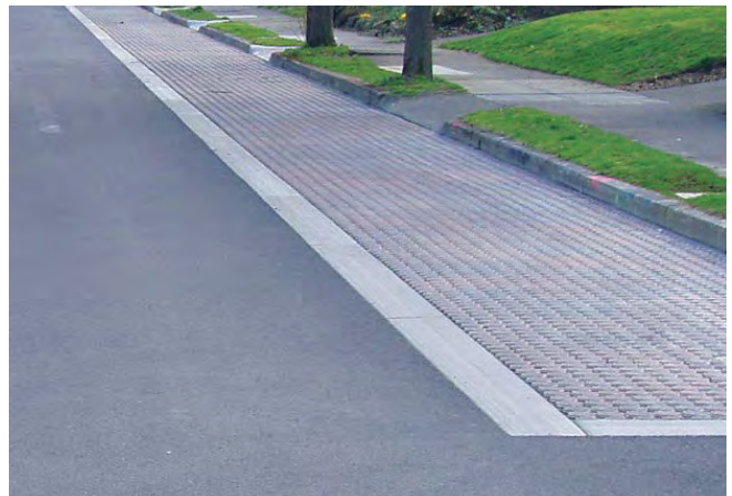
Figure X - Permeable Pavers for On-Street Parking (Source)
