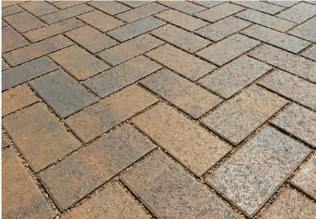
Figure X - Pervious Pavers (Source)
