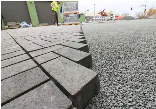
Figure X - Pervious Pavers (Source)
