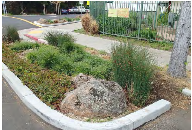
Figure X - Stormwater Bulb-Out (Source)
