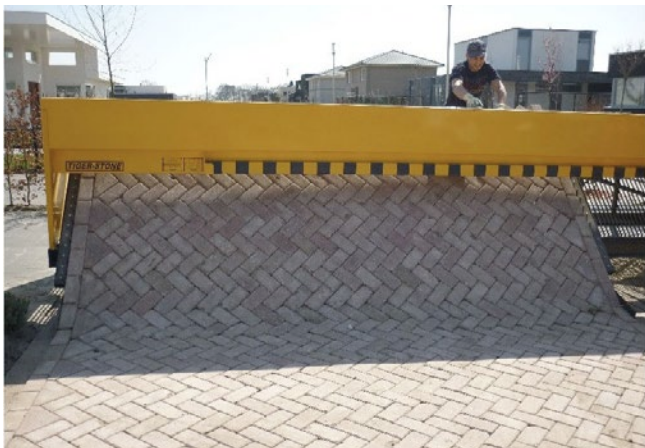
Figure X - Paver Laying Machine (Source)
