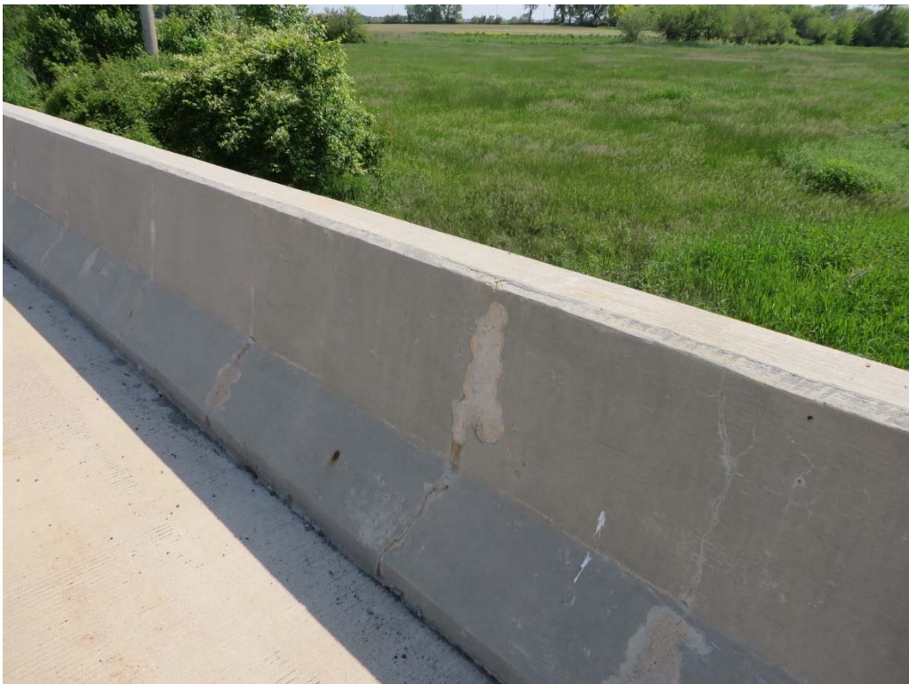
Surface Flaking on Parapet (typical)
