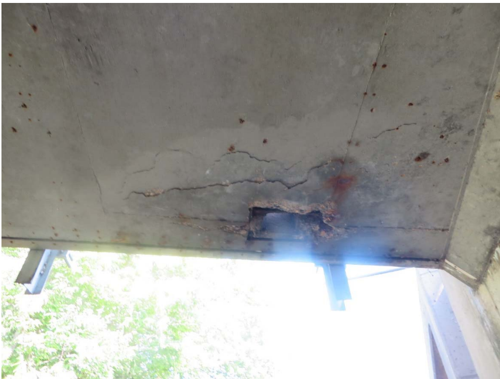
Typical Delamination Surrounding Deck Drain Opening
