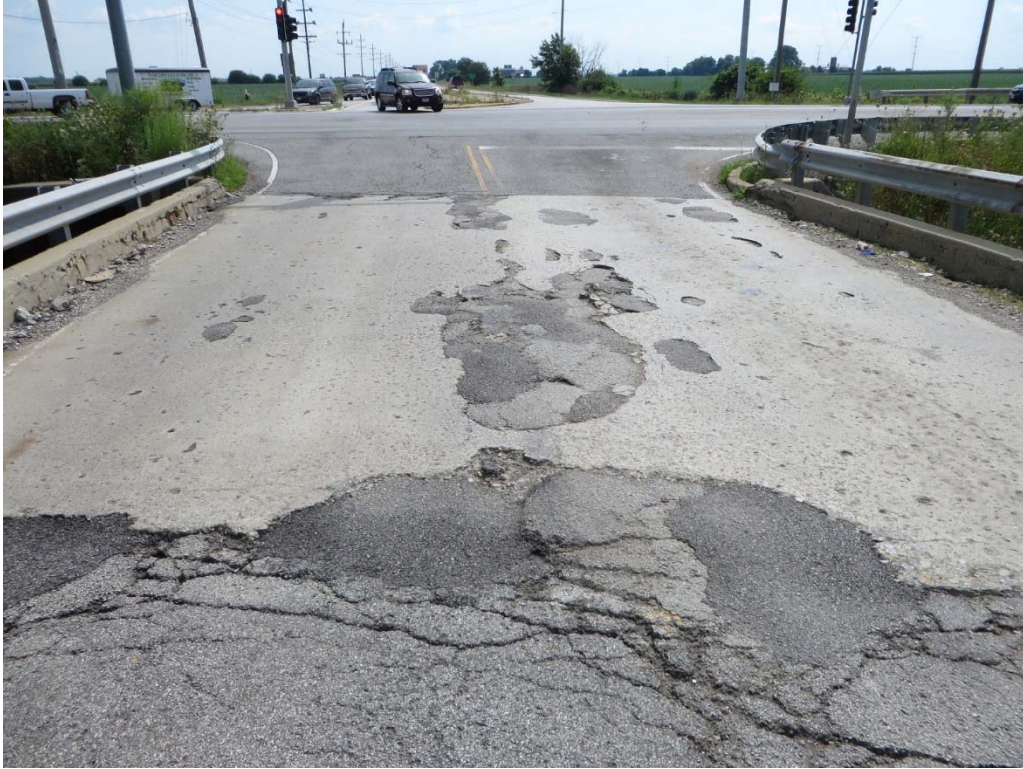
Top of Deck Showing Spalls with Failing Patches
