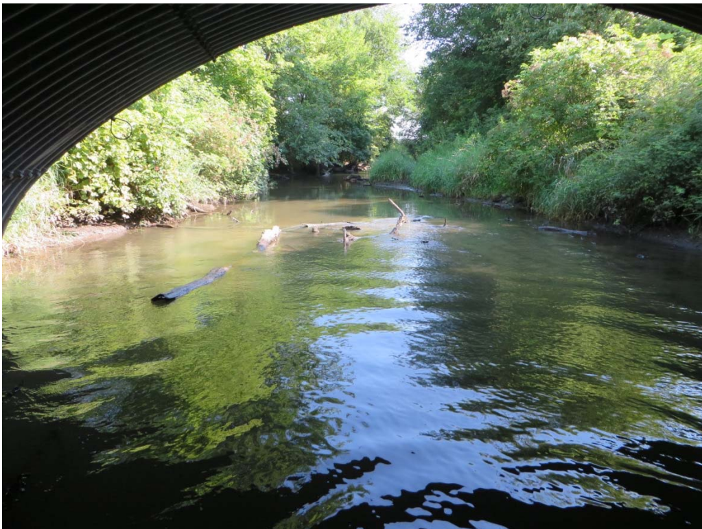
Branches Impeding Flow just Upstream (North) of Culvert
