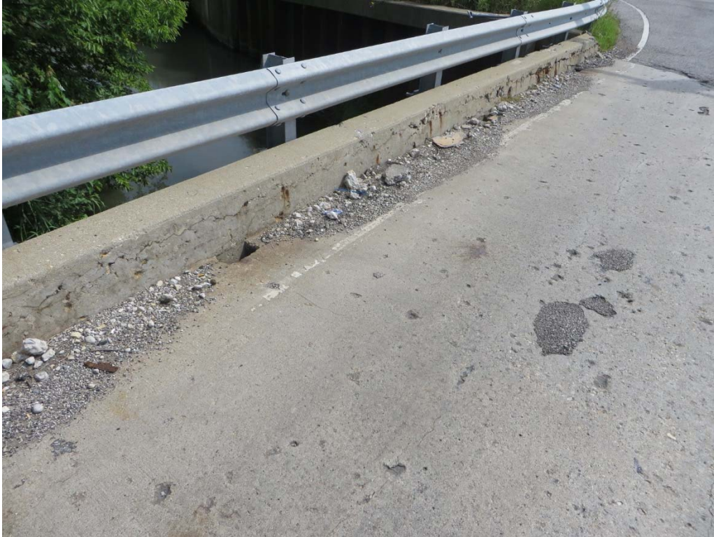
Debris, Spalls with Exposed Rebar and Delaminations in North Curb
