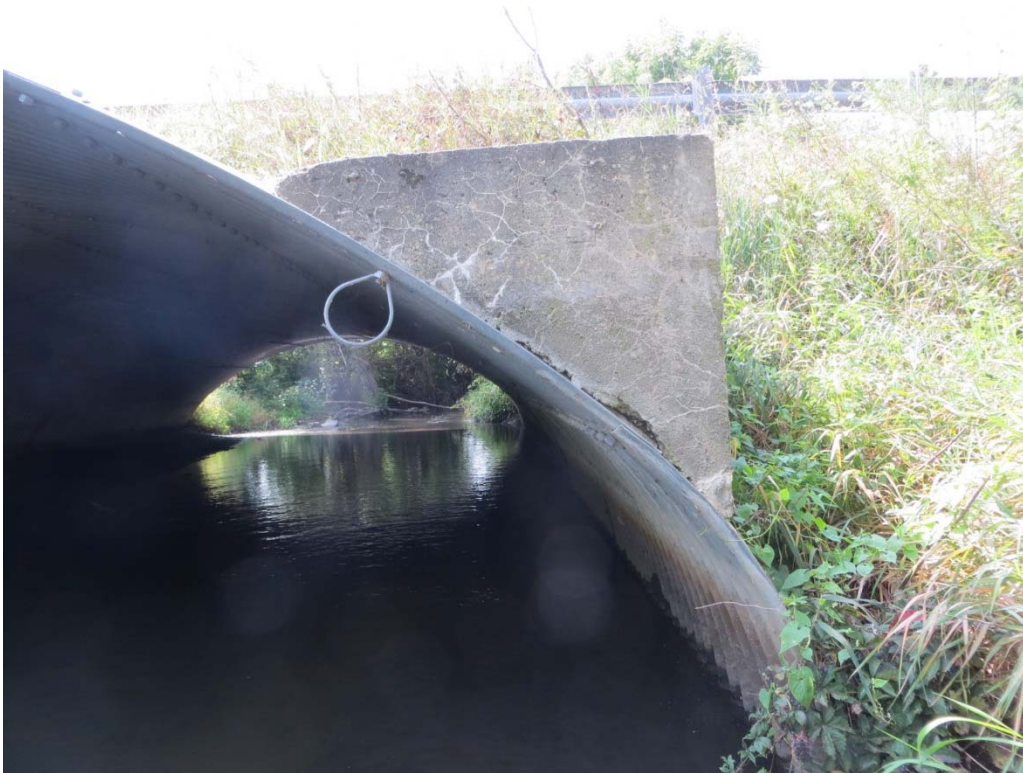
Concrete Thrust Beams Full Length of Culvert (Both Sides)
