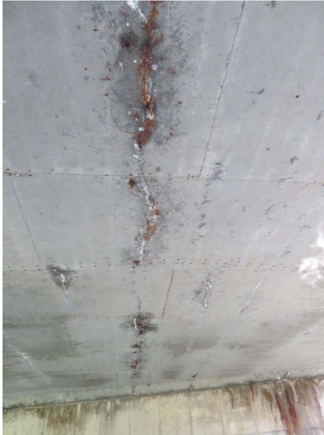
Damp Concrete and Leaching on Underside of Deck
