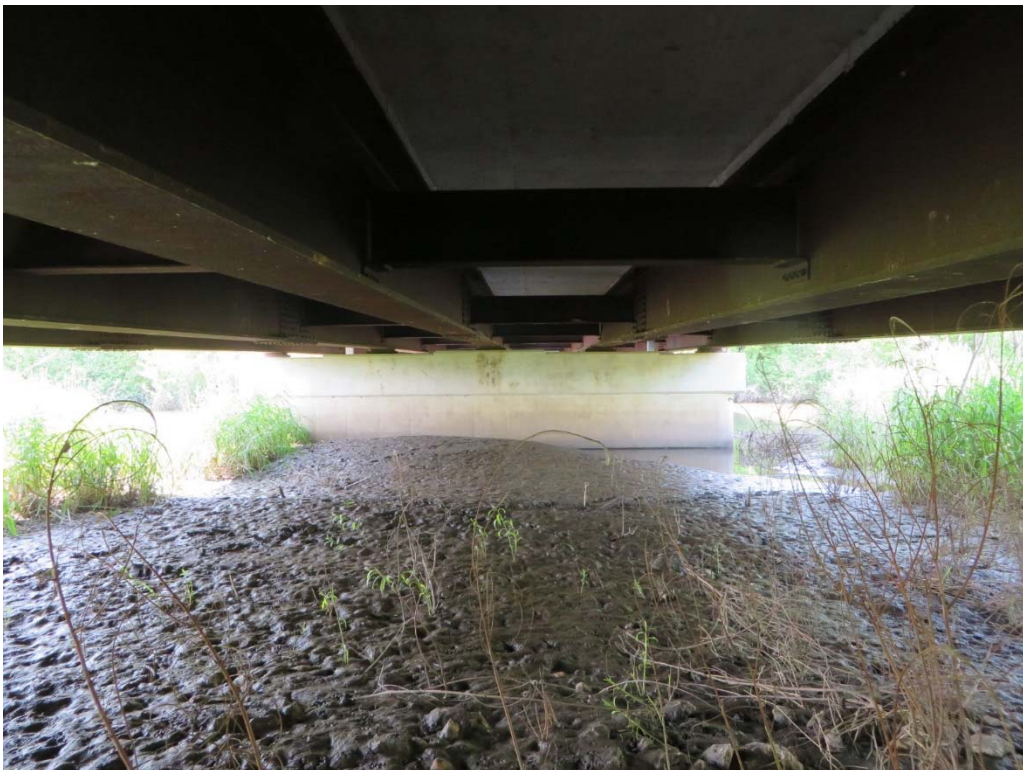
Mud Blocking Creek in South Span
