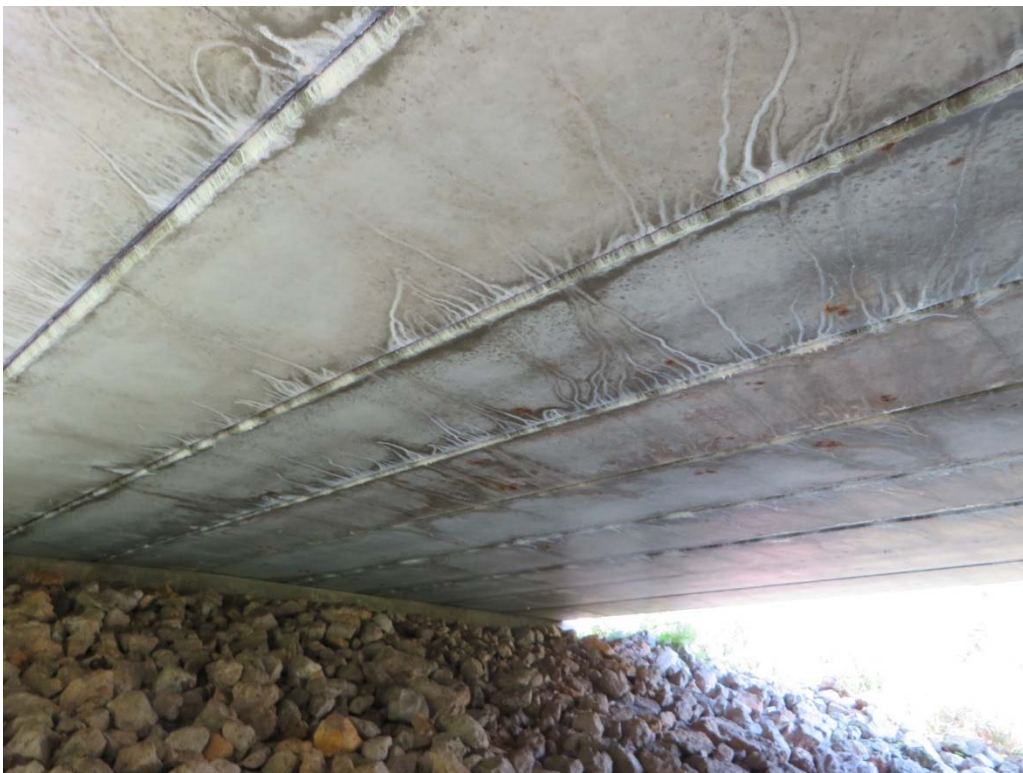
Leaching on Underside of Beams at Shear Keys
