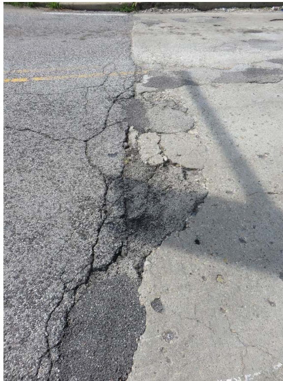
Spalls with Failing Patches at East End of Deck (West End Similar)
