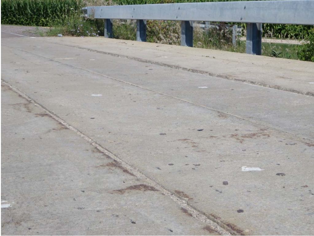
Differential Movement between Adjacent Beams
