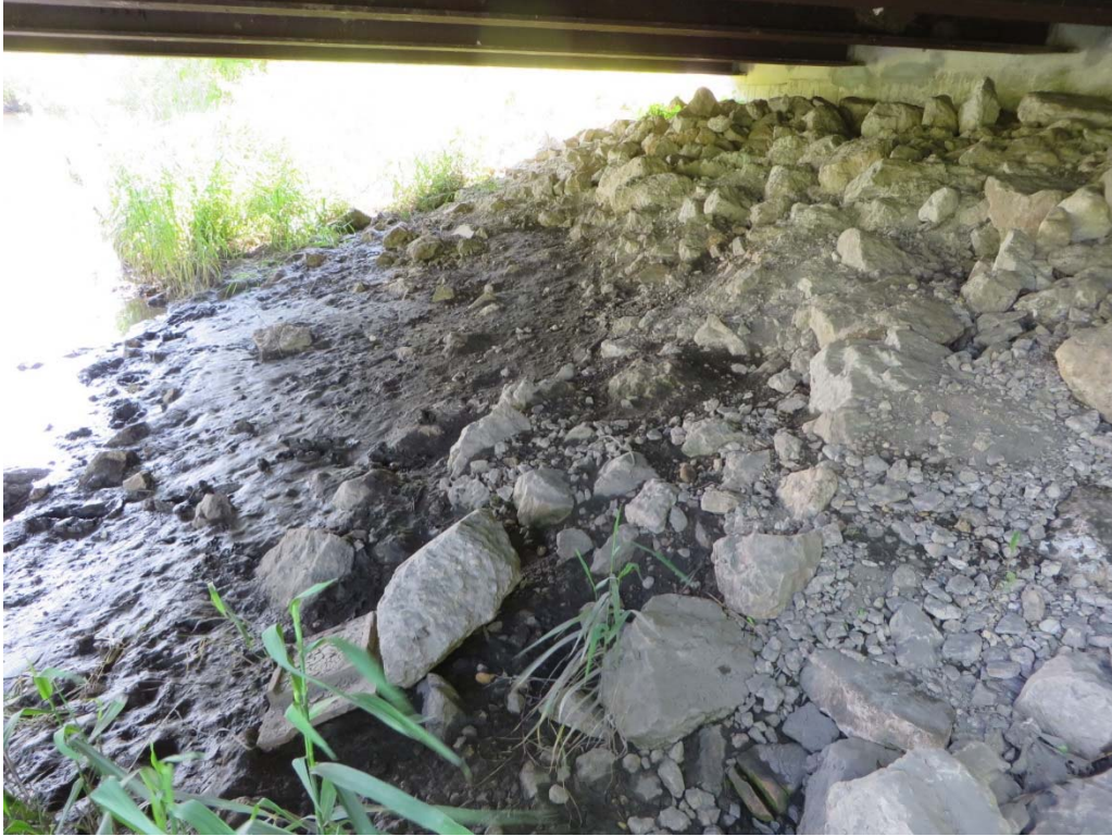
North Slopewall with Missing Riprap
