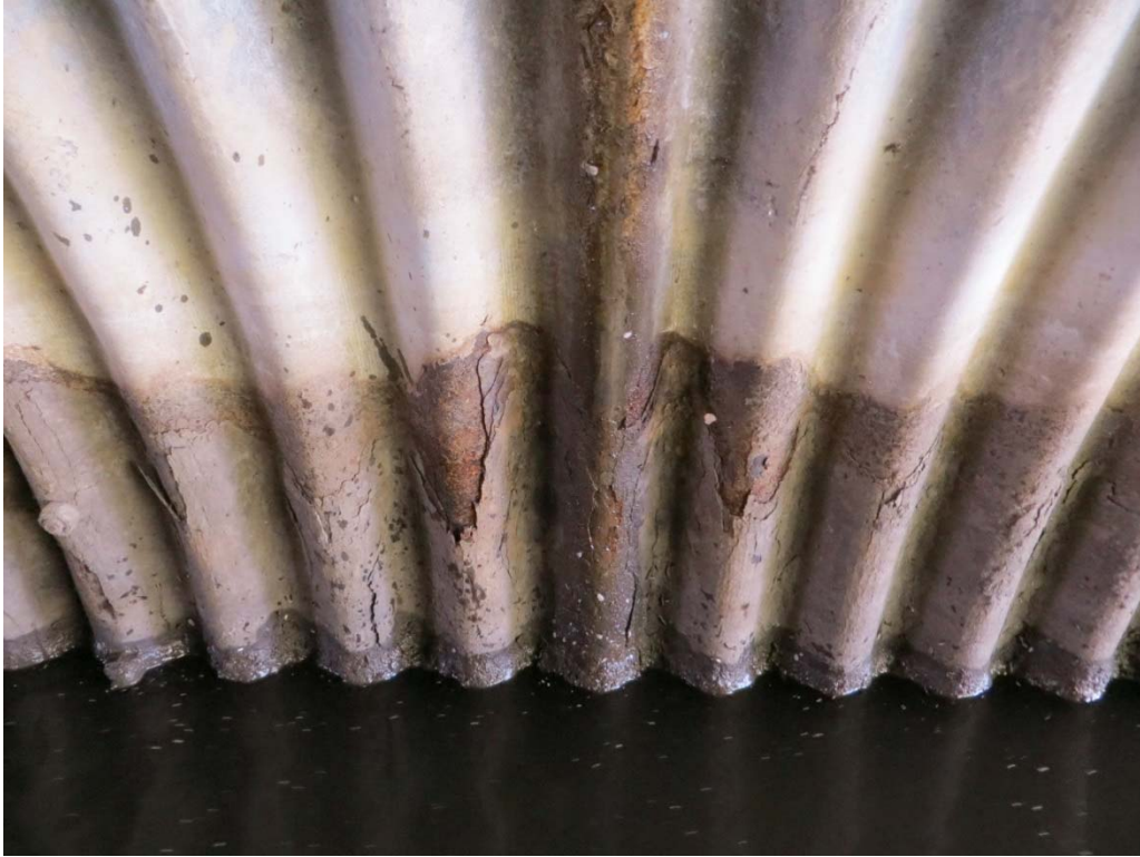
Typical Minor Section Loss at Waterline
