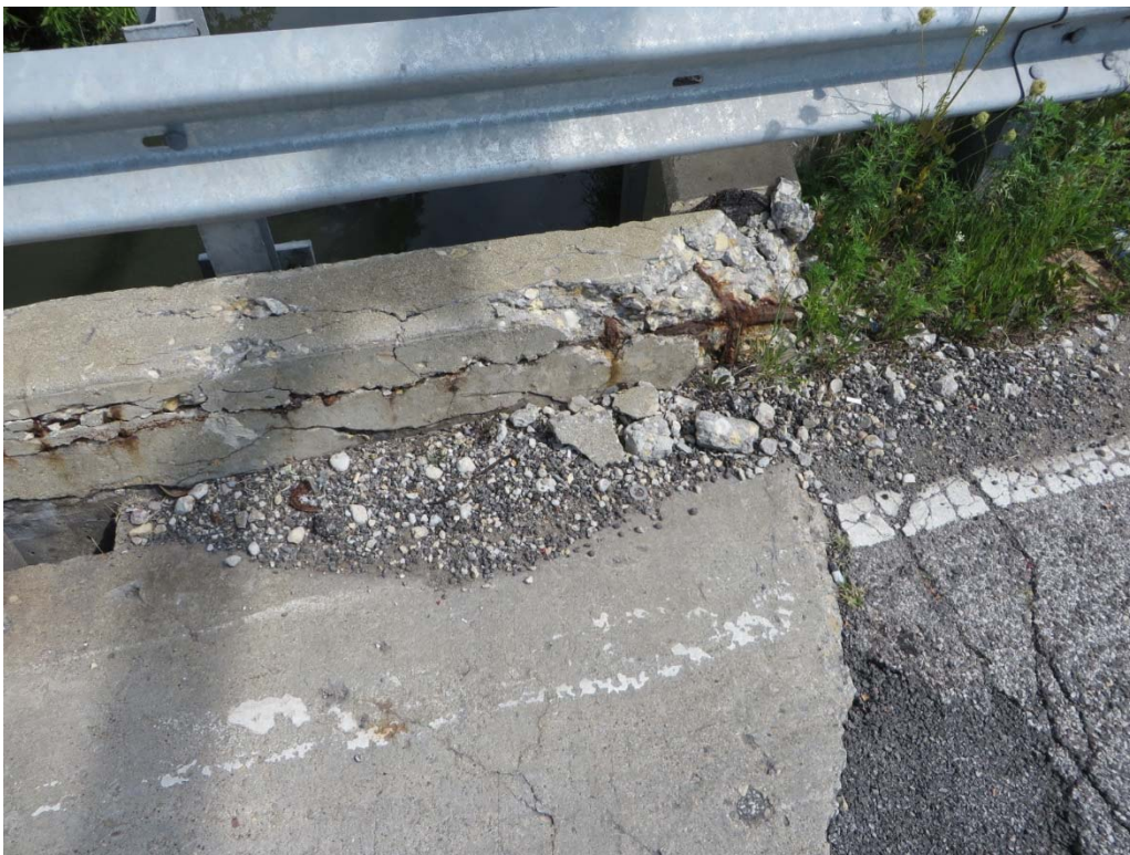
Northeast corner of Curb with Spall Exposing Rebar
