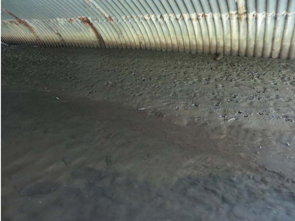
Sediment Build-up along East Edge of the Culvert
