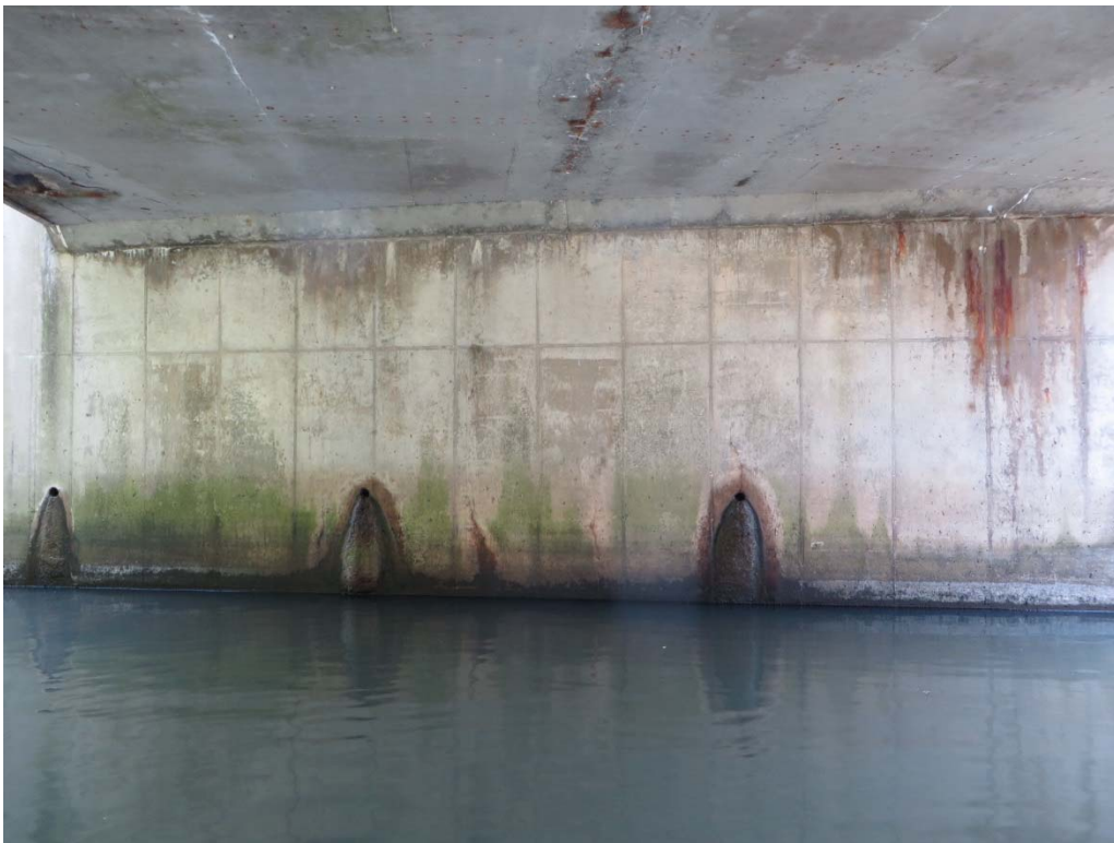
East Abutment Elevation with Dampness and Rust Stains
