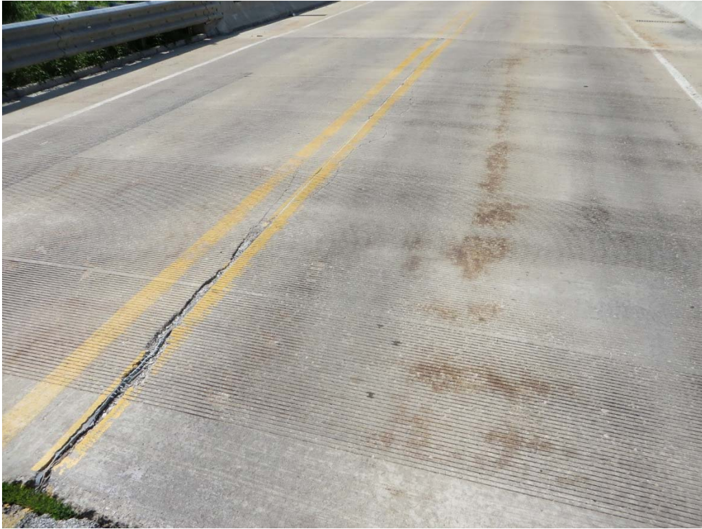
Narrow Longitudinal Cracks in South Approach Slab
