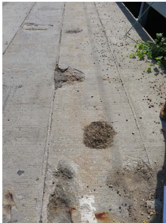
Spalls with Exposed Stirrups (SW Corner Shown)
