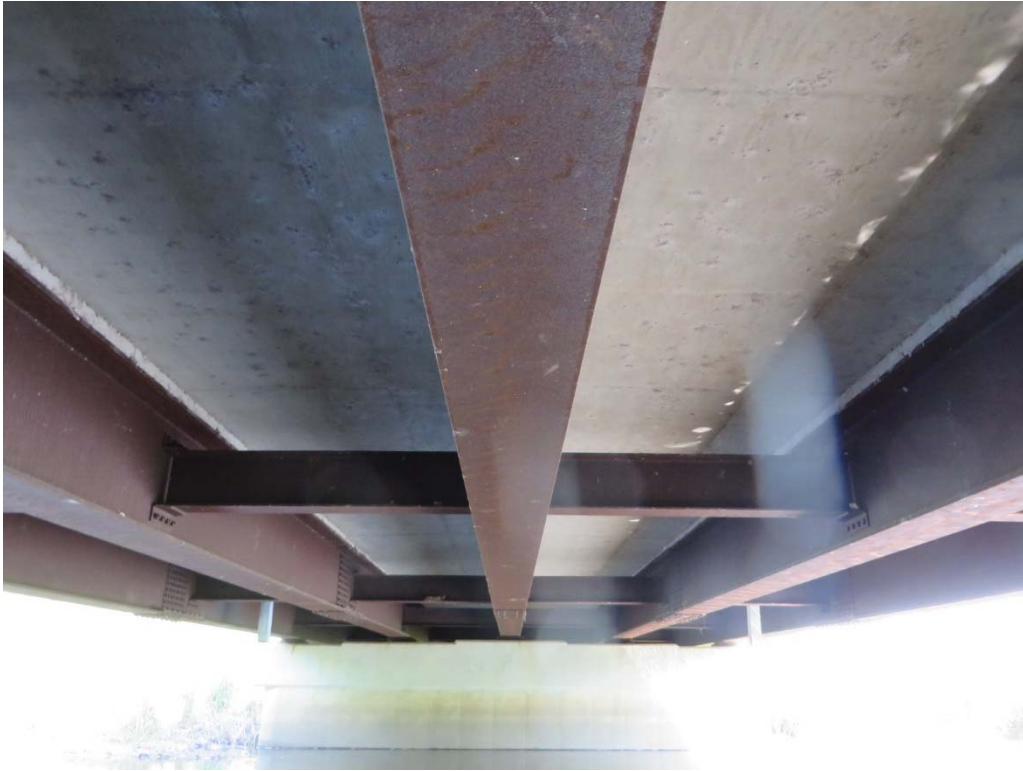
Typical Superstructure and Underside of Deck
