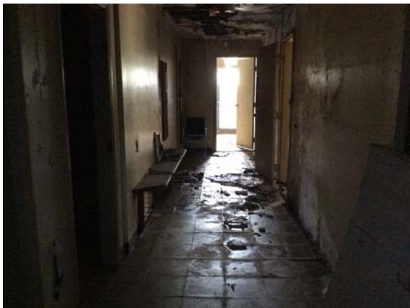
PHOTO #35: CENTRAL HALLWAY
