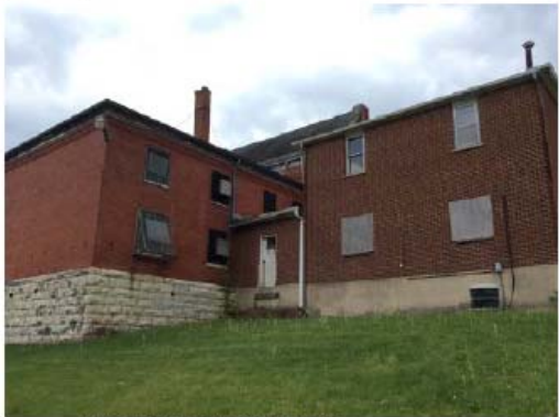
PHOTO #3: NORTH ELEVATION
