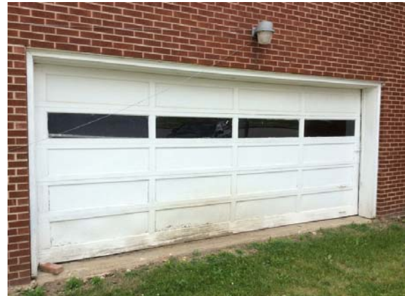
PHOTO #14: GARAGE DOOR, WOOD
