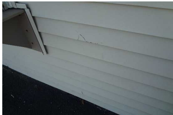
#10: DAMAGED VINYL SIDING
