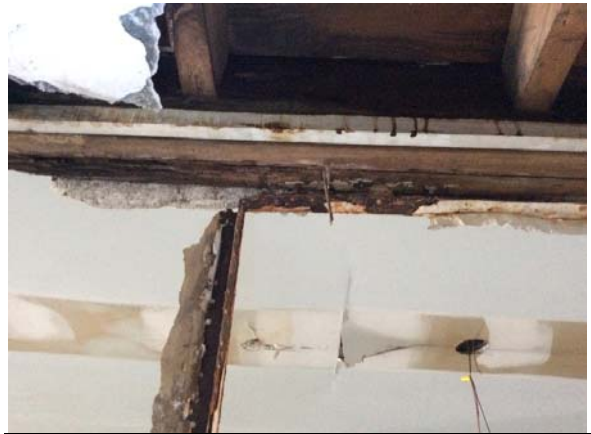
PHOTO #50: WATER DAMAGED CEILING
