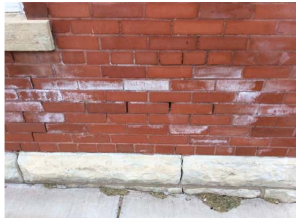
PHOTO #10: EFFLORESCENCE AND DETERIORATED MORTAR
