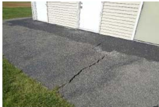
#6: PEDESTRIAN PAVEMENT, SIDEWALK, CRACKING
