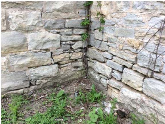
PHOTO #15: FOUNDATION WALL, MISSING MORTAR, LOOSE STONES
