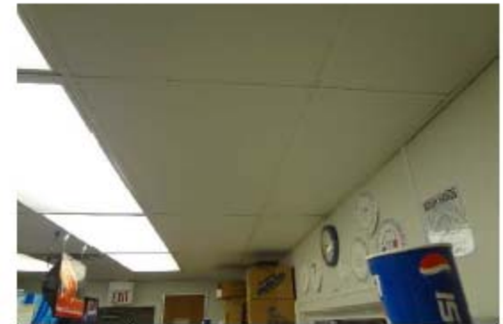
#33: INTERIOR CEILING FINISH, ACOUSTICAL TILE (ACT)
