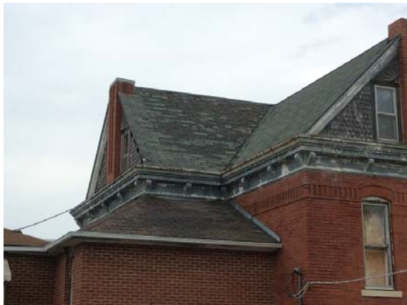
PHOTO #9: ASPHALT SHINGLE ROOF, DETERIORATING
