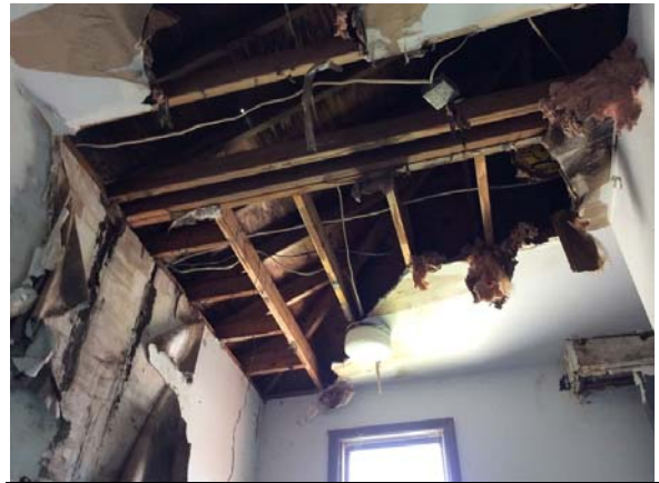
PHOTO #38: WATER DAMAGE, SECOND FLOOR, SOUTH STAIRS
