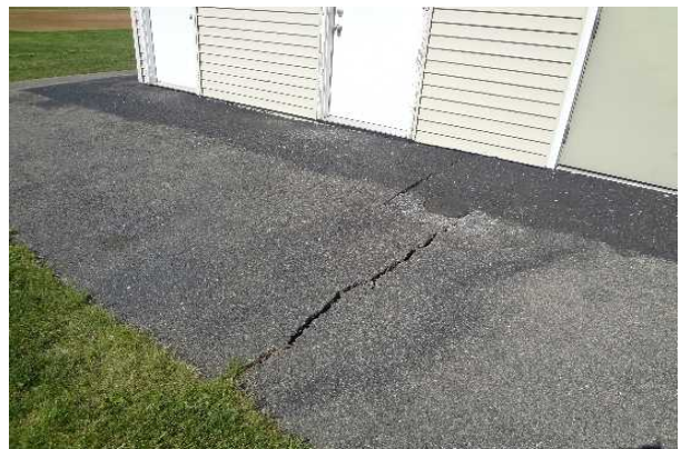
#6: PEDESTRIAN PAVEMENT, SIDEWALK, CRACKING
