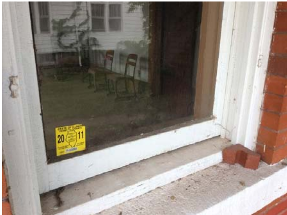
PHOTO #13: WINDOW, WOOD FRAME, SINGLE PANE
