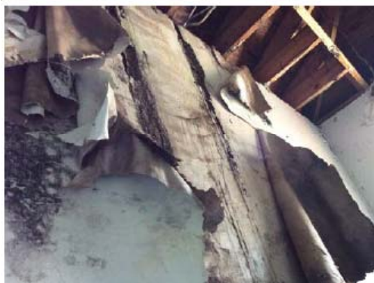
PHOTO #39: WATER DAMAGE
