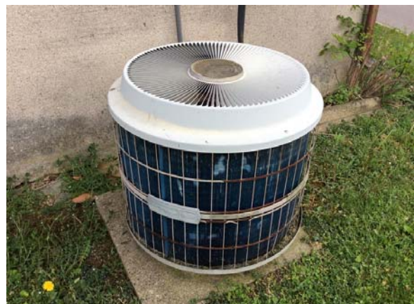
PHOTO #18: CONDENSING UNIT
