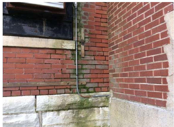
PHOTO #12: MISSING MORTAR
