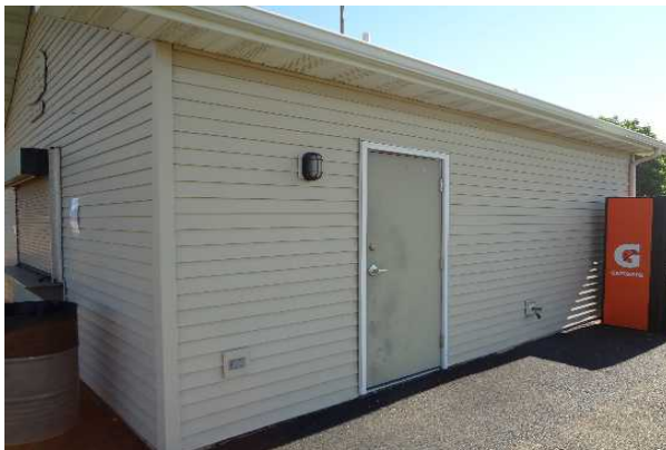
#9: EXTERIOR WALL, VINYL SIDING
