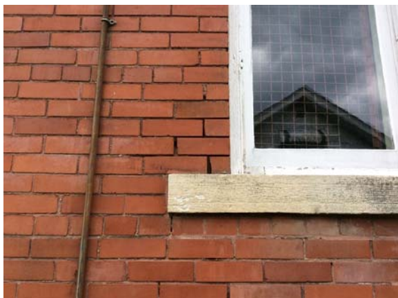
PHOTO #11: MISSING MORTAR
