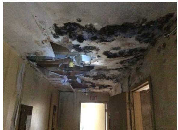
PHOTO #36: WATER DAMAGE, CENTRAL HALLWAY
