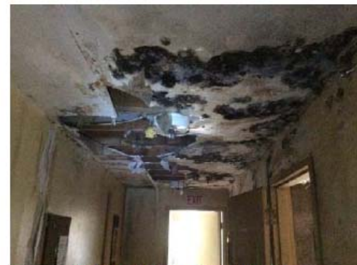
PHOTO #36: WATER DAMAGE, CENTRAL HALLWAY
