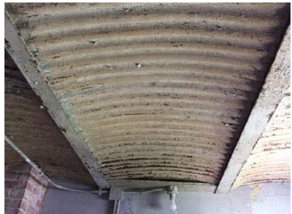
PHOTO #60: CORRUGATED STEEL ARCH FIRST FLOOR FRAMING
