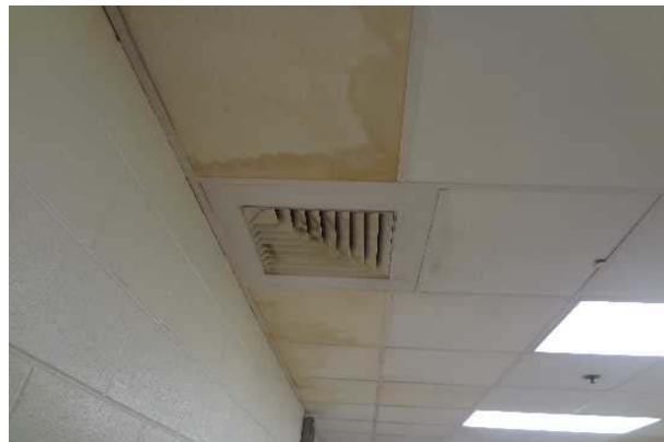
#46: WATER STAINED ACOUSTICAL TILES
