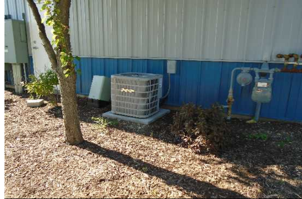
#20: CONDENSING UNIT/HEAT PUMP, SPLIT SYSTEM
