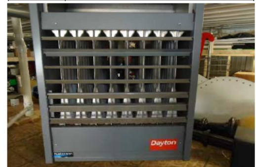
#21: UNIT HEATER, NATURAL GAS
