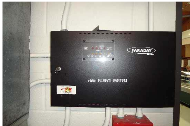
#34: FIRE ALARM CONTROL PANEL, ADDRESSABLE
