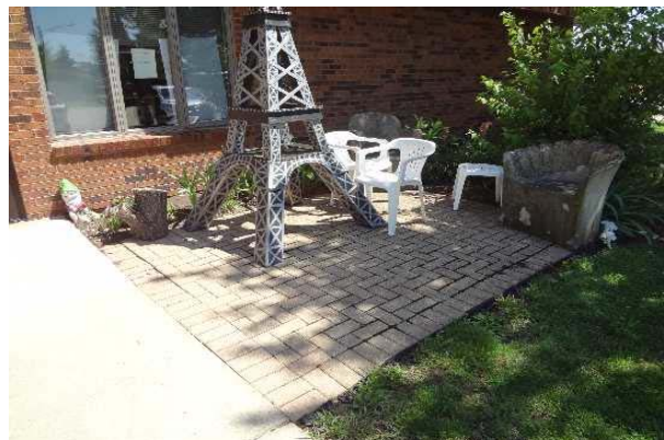
#18: PEDESTRIAN PAVEMENT, SIDEWALK, CLAY BRICK/MASONRY PAVERS
