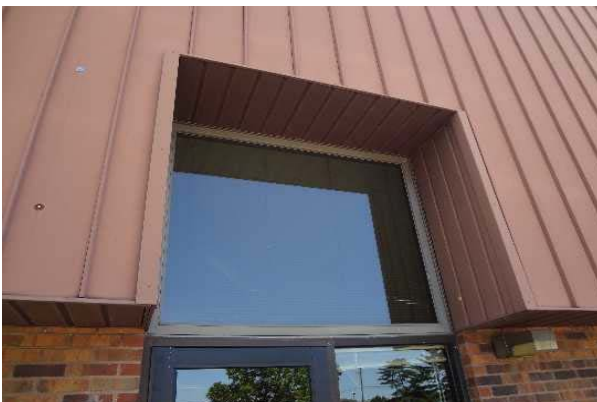
#17: WINDOW, ALUMINUM DOUBLE-GLAZED FIXED
