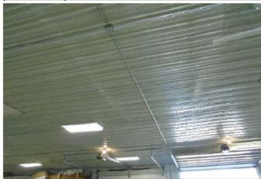
#45: INTERIOR CEILING FINISH, METAL
