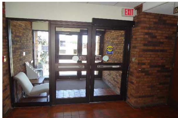
#48: INTERIOR DOOR, FULLY- GLAZED ALUMINUM-FRAMED SWINGING
