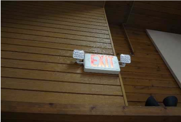
#31: EMERGENCY/EXIT LIGHT COMBO
