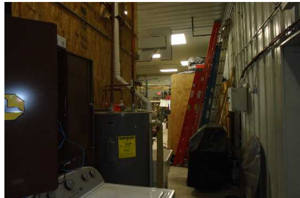
#22: WATER HEATER, ELECTRIC, RESIDENTIAL
