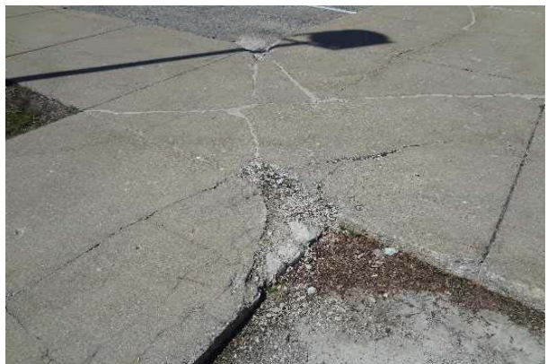
#6: DETERIORATING SIDEWALK AND REPAIRED CRACKS
