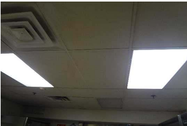
#45: INTERIOR CEILING FINISH, ACOUSTICAL TILE (ACT)
