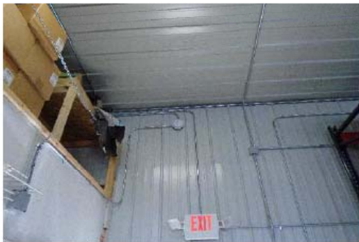
#42: INTERIOR WALL FINISH, STEEL
