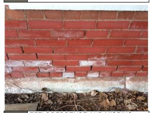
EFFLORESCENCE AND MISSING Рното **MORTAR** #16:
