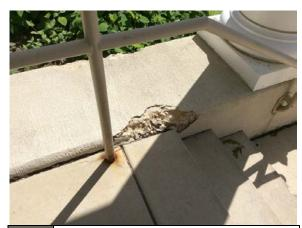
PHOTO #13: STAIR WALL, SPALLING
