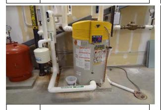
WATER HEATER, CONDENSING #47: STYLE, HIGH EFFICIENCY
