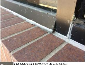
PHOTO DAMAGED WINDOW FRAME #23:
