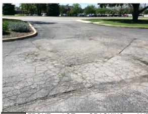
PHOTO #14: FRONT LOT, CRACKING AND DETERIORATED
