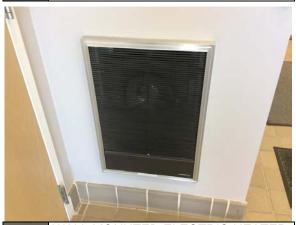
PHOTO #39: WALL MOUNTED ELECTRIC HEATER
