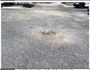
PHOTO #15: NORTHEAST LOT, CRACKING
