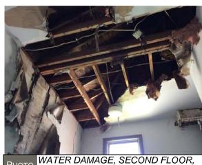
PHOTO #38: WATER DAMAGE, SECOND FLOOR, SOUTH STAIRS
