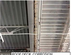
ROOF DECK, CORROSION Рното #42:
