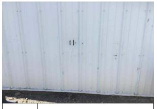
PUNCTURE TO ALUMINUM #19: SIDING ON NORTH ELEVATION OF BUILDING
