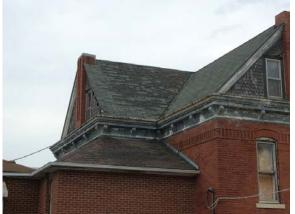
PHOTO ASPHALT SHINGLE ROOF, **DETERIORATING**
