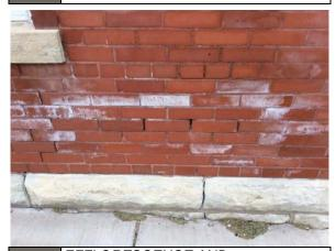
EFFLORESCENCE AND Рното DETERIORATED MORTAR #10:
