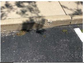
PHOTO CURB, DAMAGED #9:
