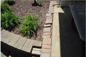
CLAY BRICK/MASONRY PAVERS, MISSING AND #12: **DISLODGED BRICKS**
