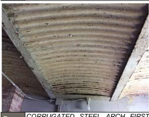
PHOTO #60: CORRUGATED STEEL ARCH FIRST FLOOR FRAMING
