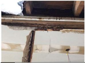
PHOTO #50: WATER DAMAGED CEILING
