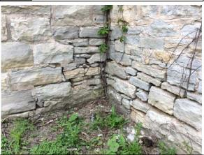
FOUNDATION WALL, MISSING MORTAR, LOOSE STONES
