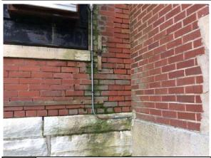
PHOTO MISSING MORTAR #12:
