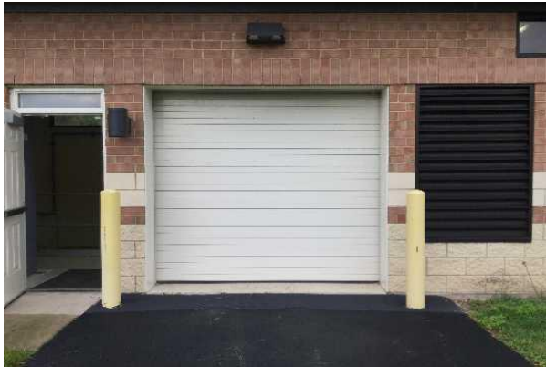
#13: OVERHEAD DOOR, ALUMINUM ROLL-UP
