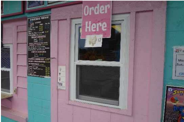
#14: WINDOW, VINYL-CLAD DOUBLE-GLAZED 6 SF
