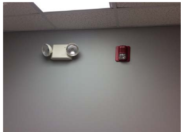
PHOTO #40: BACKUP LIGHT FIXTURE AND STROBE ALARM
