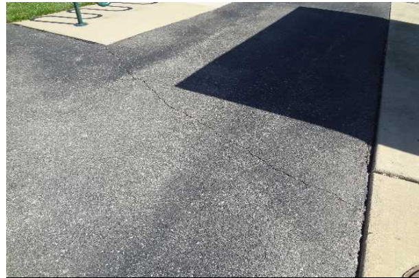
#4: SIDEWALK, MINOR CRACKING
