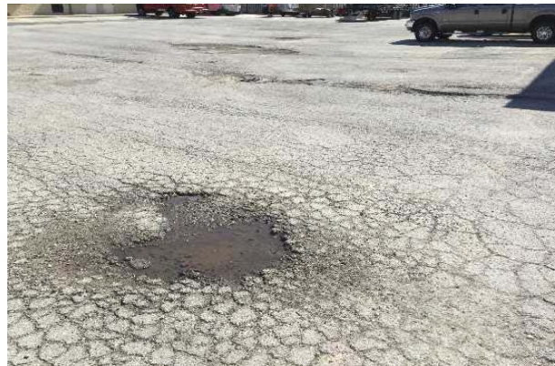
#10: PARKING LOTS, CRACKING IN ASPHALT
