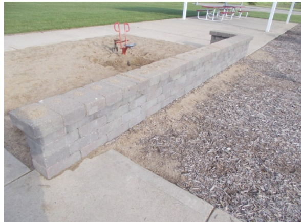
PHOTO #24: CMU RETAINING WALL
