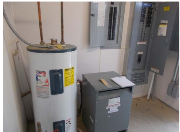
PHOTO #34: ELECTRIC WATER HEATER
