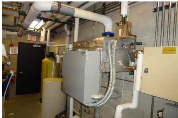
#36: HUMIDIFIER, STEAM, DUCT W/ CONTROLS
