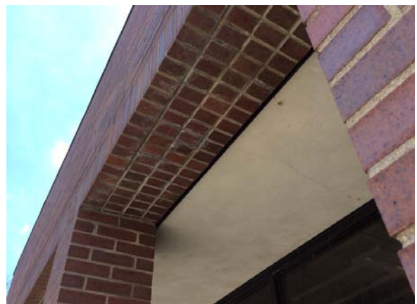
PHOTO #24: EFFLORESCENCE ON BRICK
