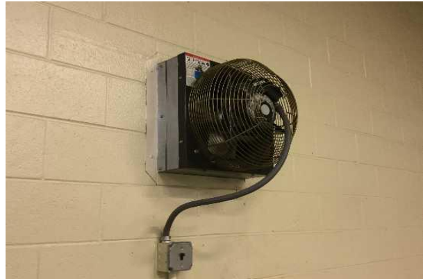
#14: EXHAUST FAN, PROPELLER
