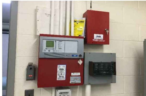
#40: FIRE ALARM CONTROL PANEL, ADDRESSABLE
