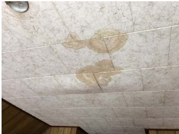
PHOTO #57: WATER DAMAGE, THIRD FLOOR
