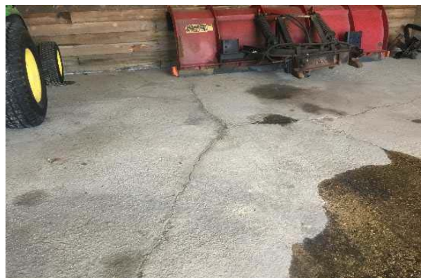
#6: CRACKING THROUGHOUT CONCRETE SLAB-ON-GRADE
