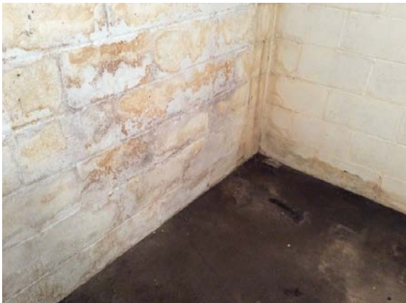
PHOTO #59: EFFLORESCENCE AND WATER STAINING
