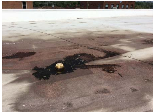
PHOTO #26: ROOF, WATER STAINING
