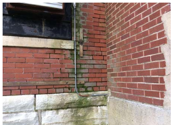
PHOTO #12: MISSING MORTAR
