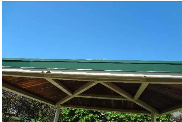
#16: CHIPPED PAINT AND CORROSION
