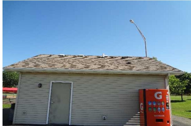
#8: ROOF, ASPHALT SHINGLE
