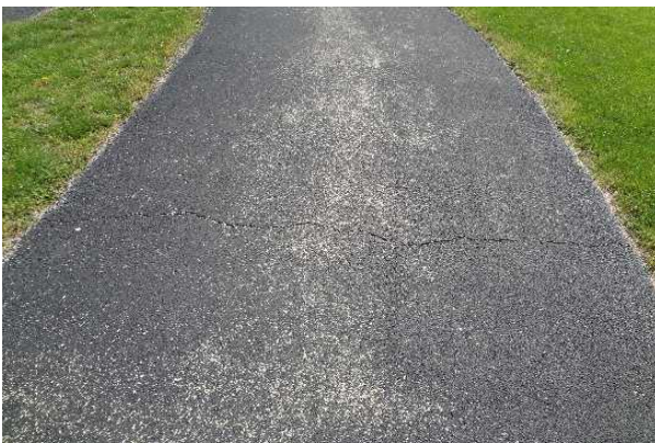
#5: PEDESTRIAN PAVEMENT, MINOR CRACKING
