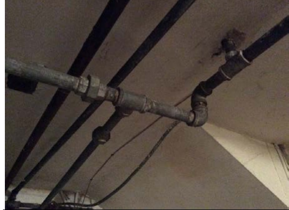
PHOTO #28: GALVANIZED WATER PIPE
