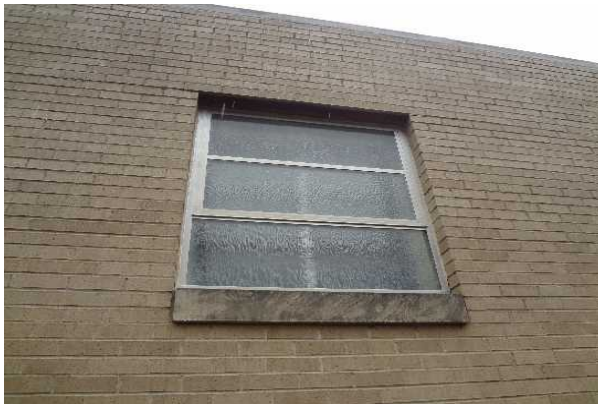
#15: WINDOW, ALUMINUM DOUBLE-GLAZED AWNING
