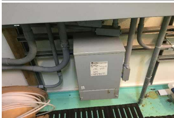
#17: SECONDARY TRANSFORMER, DRY
