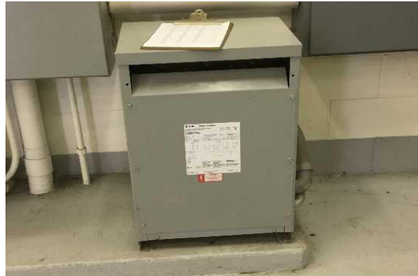
#26: SECONDARY TRANSFORMER
