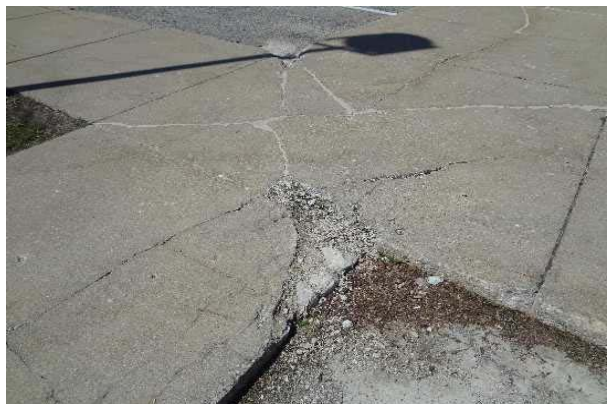
#6: DETERIORATING SIDEWALK AND REPAIRED CRACKS
