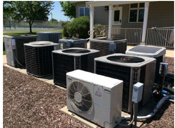
PHOTO #32: CONDENSING UNITS
