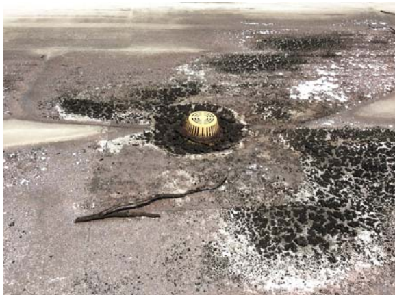
PHOTO #27: ROOF, CLOGGED DRAIN
