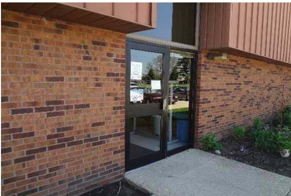
#15: EXTERIOR DOOR, FULLY-GLAZED ALUMINUM-FRAMED SWINGING
