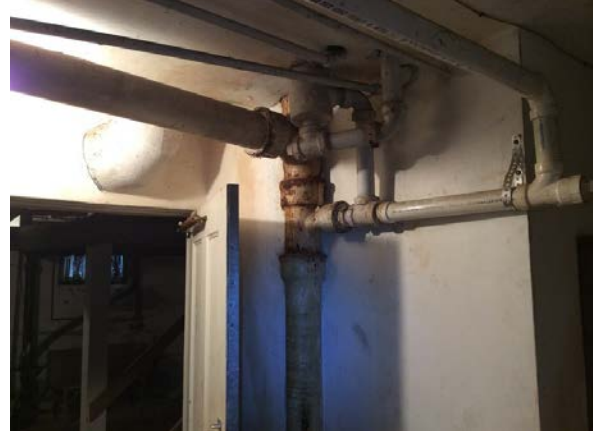
PHOTO #30: CAST IRON SANITARY PIPE, AGED
