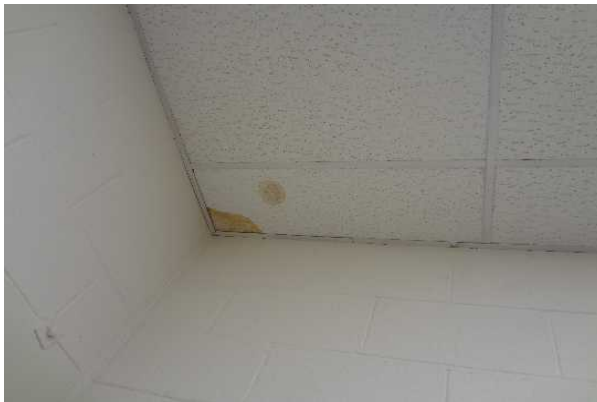
#39: STAINED ACOUSTICAL CEILING TILE
