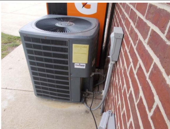
PHOTO #29: CONDENSING UNIT
