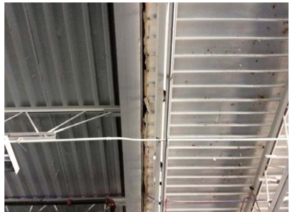
PHOTO #42: ROOF DECK, CORROSION
