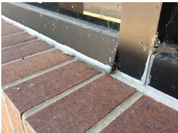
PHOTO #23: DAMAGED WINDOW FRAME
