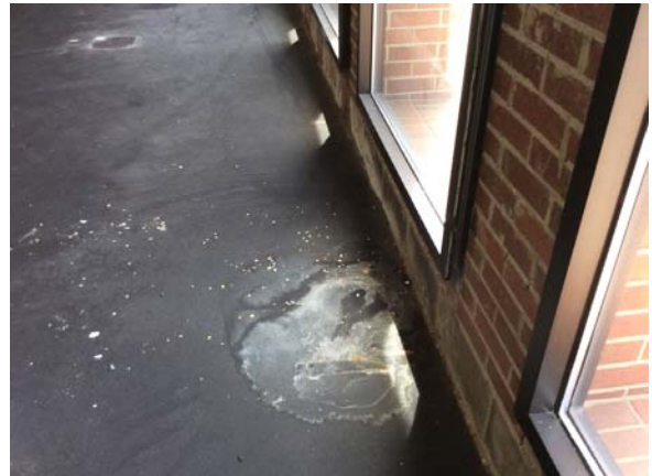
PHOTO #44: WATER STAIN ADJACENT TO EAST WALL
