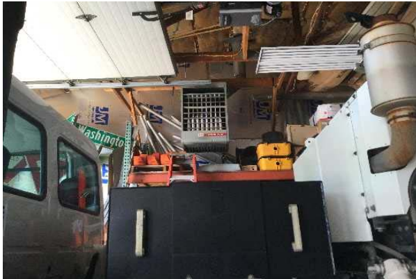
#13: UNIT HEATER, NATURAL GAS
