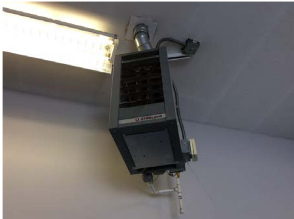
PHOTO #37: UNIT HEATER, SALLY PORT
