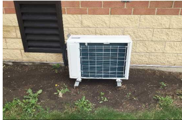
#14: DUCTLESS SPLIT SYSTEM, SINGLE ZONE
