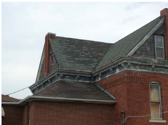
PHOTO #9: ASPHALT SHINGLE ROOF, DETERIORATING
