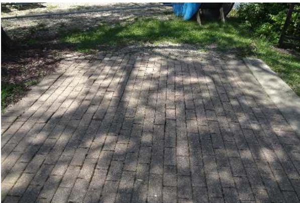
#5: SIDEWALK, DISPLACED PAVERS
