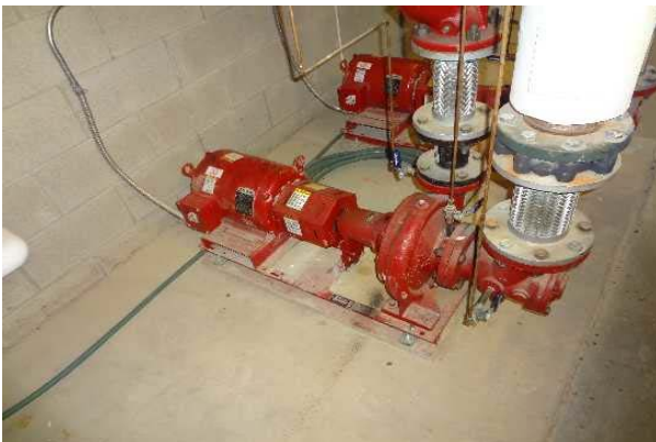
#35: CIRCULATION PUMP, HEATING WATER, SECONDARY
