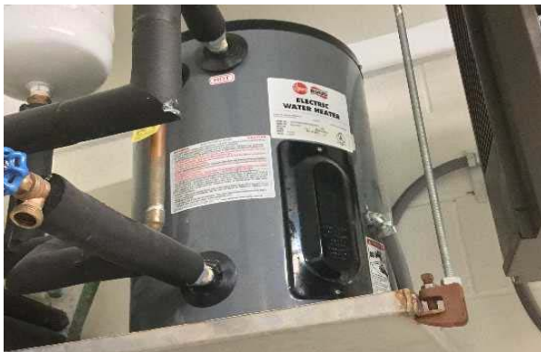
#27: WATER HEATER, ELECTRIC, RESIDENTIAL
