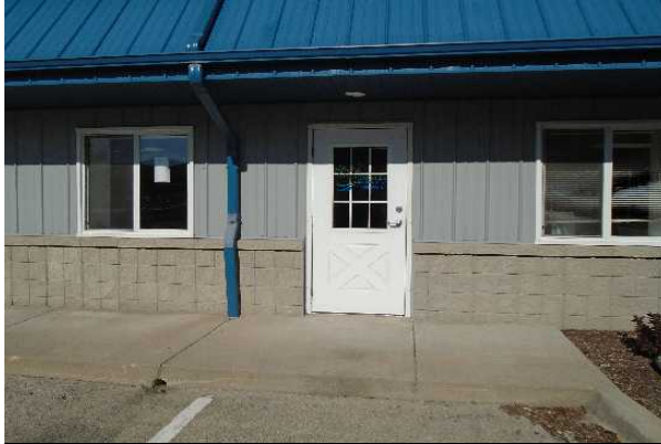
#13: EXTERIOR DOOR, STEEL W/ GLASS
