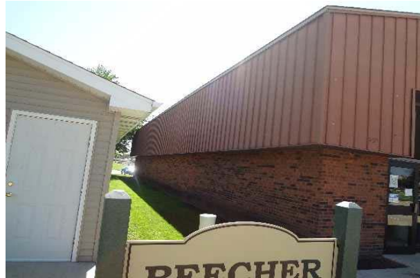
#14: EXTERIOR WALL, ALUMINUM SIDING
