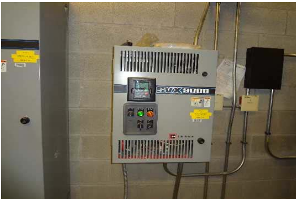
#57: VARIABLE FREQUENCY DRIVE (VFD)
