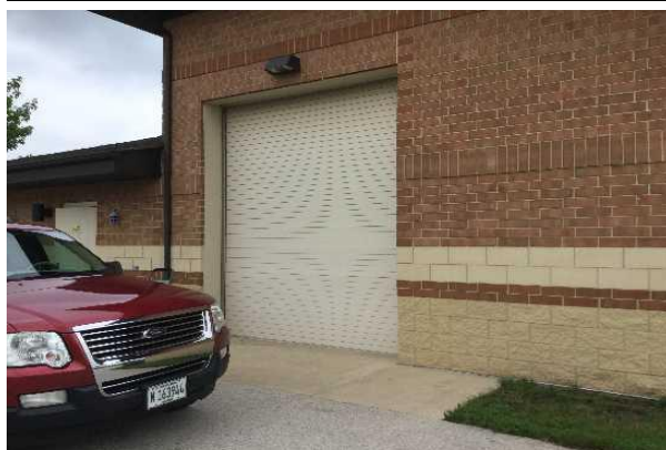
#11: OVERHEAD DOOR, ALUMINUM ROLL-UP
