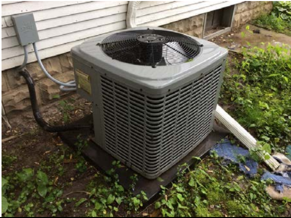
PHOTO #25: CONDENSING UNIT
