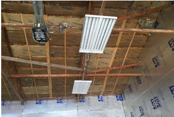
#19: 8-BULB FLUORESCENT LIGHTING FIXTURE, HIGH BAY
