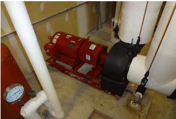
#33: CIRCULATION PUMP, CHILLER WATER
