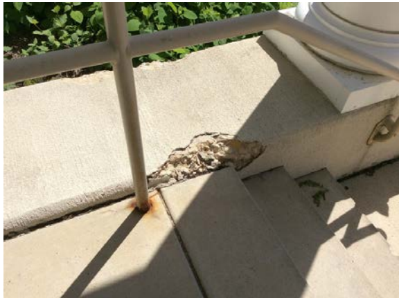
PHOTO #13: STAIR WALL, SPALLING
