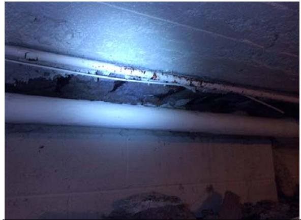
PHOTO #62: DETERIORATING CONCRETE
