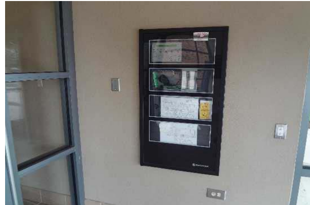
#68: FIRE ALARM CONTROL PANEL, ADDRESSABLE
