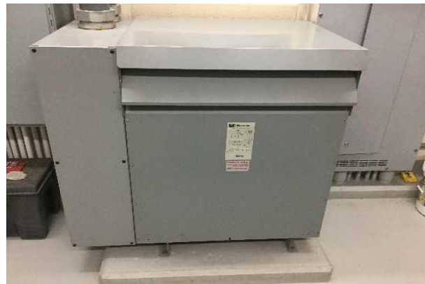
#34: SECONDARY TRANSFORMER, DRY
