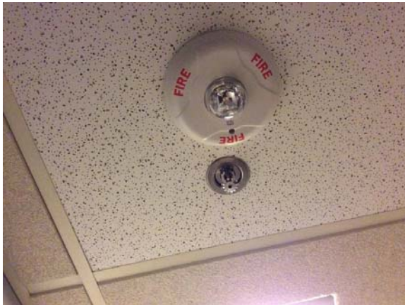
PHOTO #49: FIRE ALARM STROBE AND SPRINKLER HEAD
