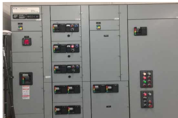
#30: MOTOR CONTROL CENTER W/ MAIN BREAKER
