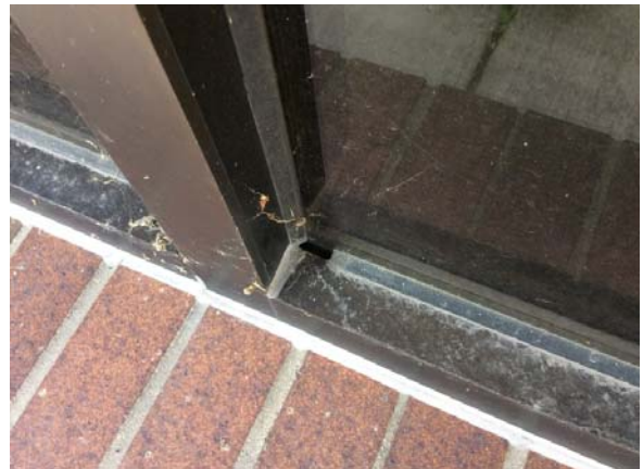
PHOTO #22: MISSING AREA OF WINDOW GASKET
