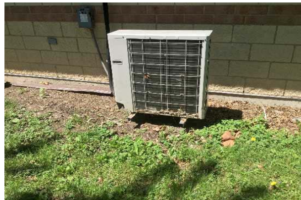
#16: DUCTLESS SPLIT SYSTEM, SINGLE ZONE
