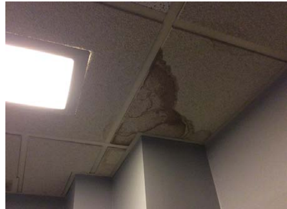
PHOTO #52: WATER DAMAGED CEILING TILE
