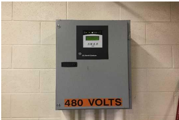
#29: AUTOMATIC TRANSFER SWITCH
