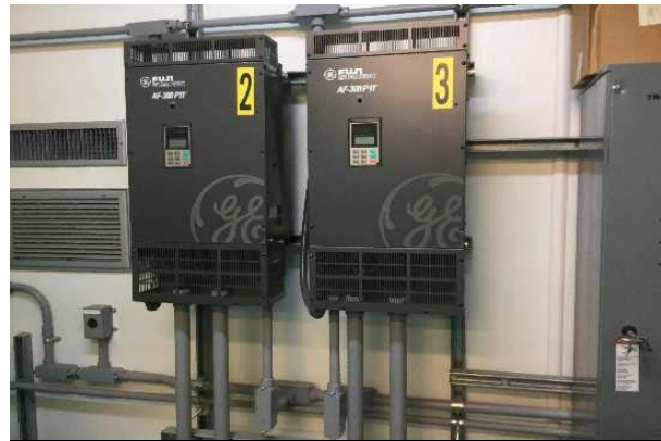
#14: VARIABLE FREQUENCY DRIVE (VFD)
