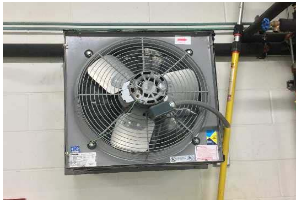
#19: EXHAUST FAN, PROPELLER
