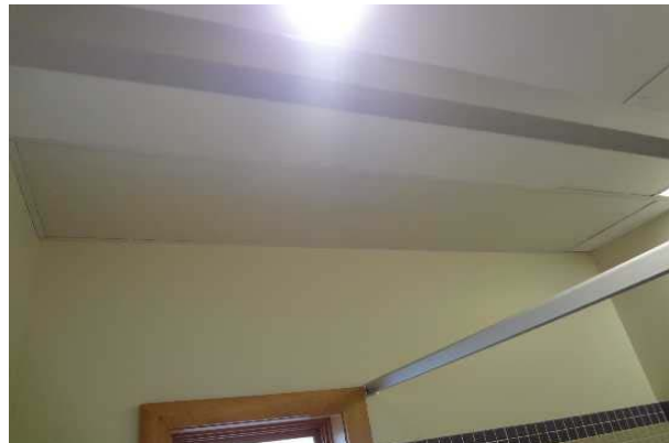
#28: RADIANT CEILING PANELS
