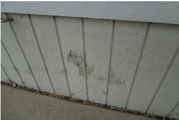
#15: EXTERIOR WALL, DAMAGED CLAPBOARD
