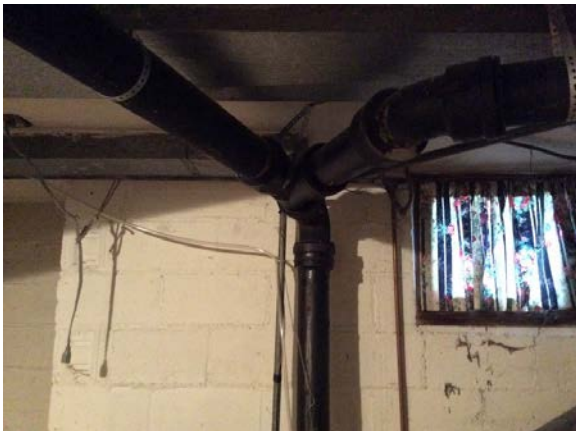
PHOTO #29: CAST IRON SANITARY PIPE
