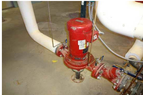
#34: CIRCULATION PUMP, HEATING WATER, PRIMARY
