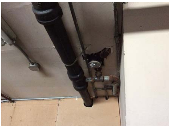
PHOTO #23: SANITARY PIPING
