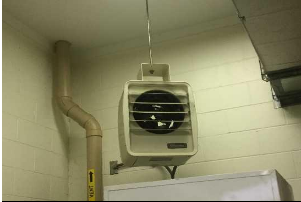
#13: UNIT HEATER, ELECTRIC
