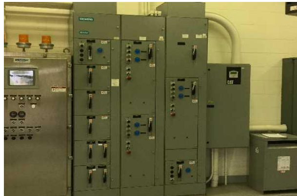
#28: MOTOR CONTROL CENTER W/ MAIN BREAKER, 3-PHASE
