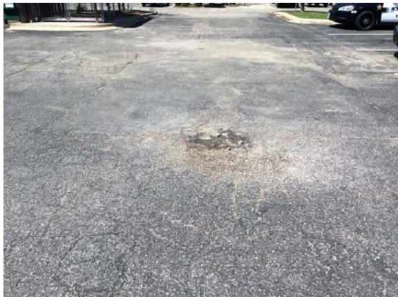
PHOTO #15: NORTHEAST LOT, CRACKING
