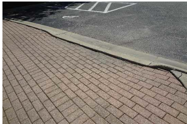
#6: SIDEWALK, DEPRESSED PAVERS
