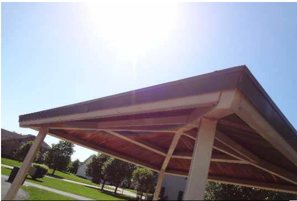
#15: STRUCTURAL FRAME, STEEL COLUMNS & BEAMS
