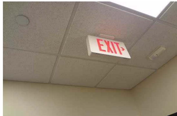
#66: EXIT LIGHTING FIXTURE, LED
