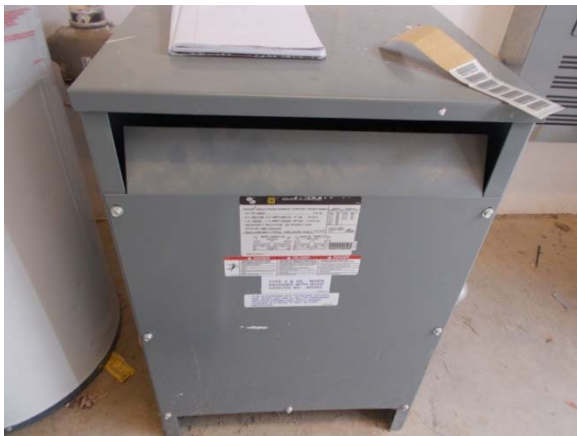
PHOTO #39: STEP DOWN TRANSFORMER
