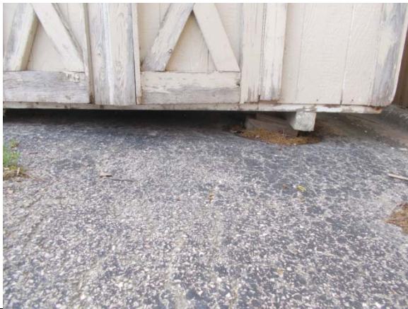
PHOTO #7: FOOTING (SUPPORT) OF SHED
