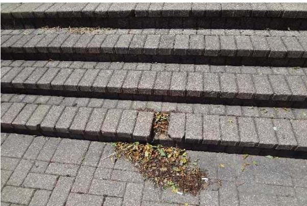
#11: STAIR, MISSING BRICK
