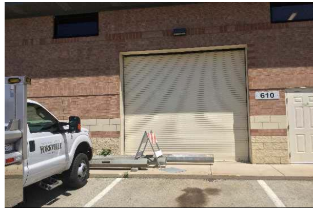
#8: OVERHEAD DOOR, ALUMINUM ROLL-UP
