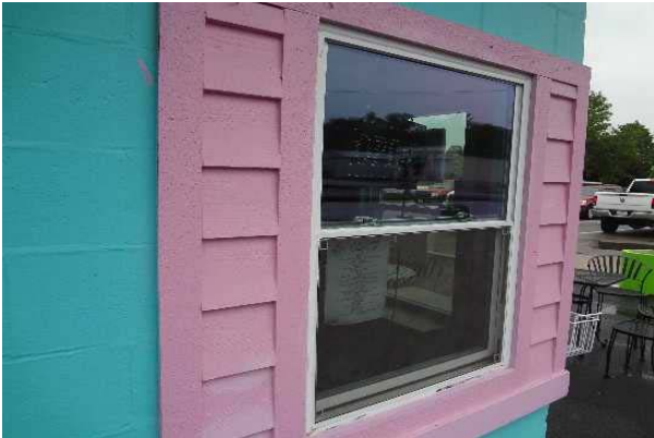
#13: WINDOW, VINYL-CLAD DOUBLE-GLAZED 12 SF
