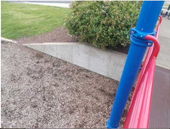
PHOTO #11: CONCRETE RETAINING WALL
