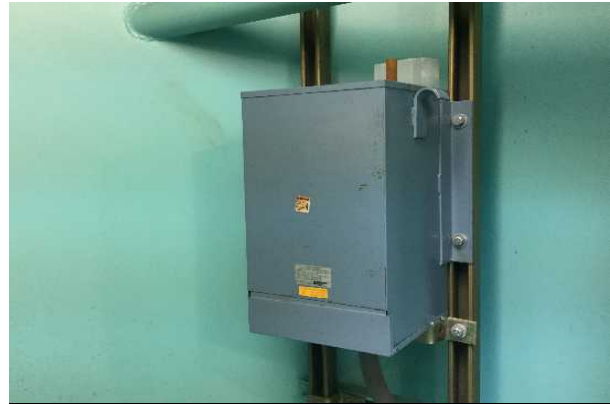
#14: SECONDARY TRANSFORMER, DRY
