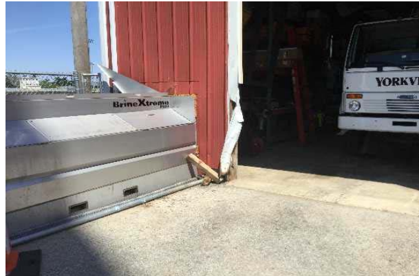
#8: SIDING PEELING OFF LEFT GARAGE ON SOUTH ELEVATION
