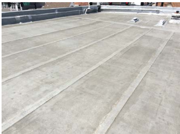
PHOTO #29: ROOF, MODIFIED BITUMINOUS MEMBRANE
