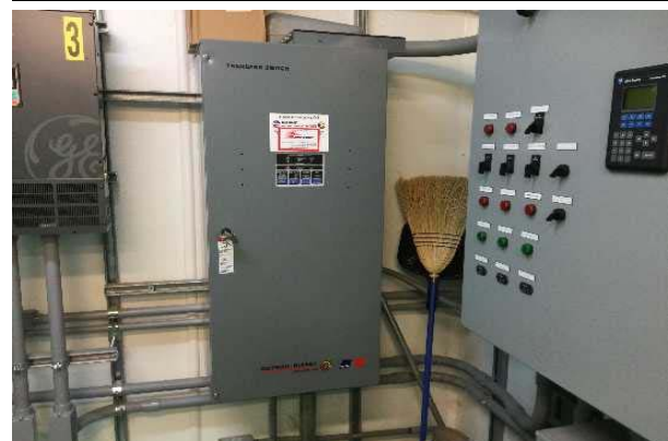
#12: TRANSFER SWITCH, AUTOMATIC (ATS)
