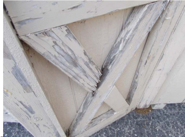
PHOTO #8: DETERIORATED DOOR
