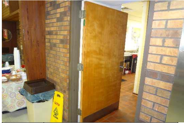
#50: INTERIOR DOOR, FIRE 90-MINUTES AND OVER
