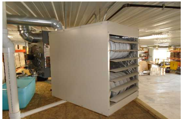
#18: UNIT HEATER, NATURAL GAS
