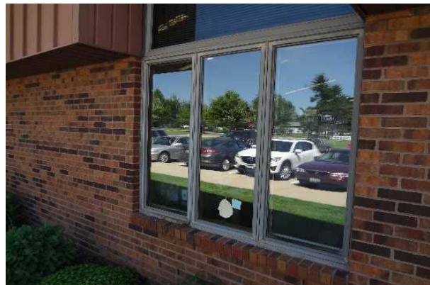
#16: WINDOW, ALUMINUM DOUBLE-GLAZED OPERABLE
