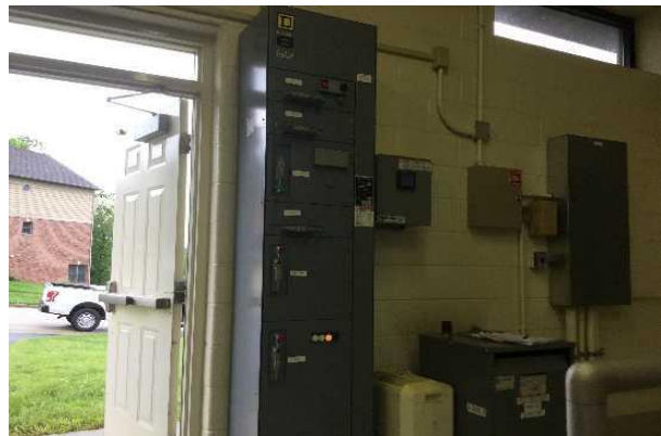
#24: MOTOR CONTROL CENTER W/ MAIN BREAKER, 3-PHASE
