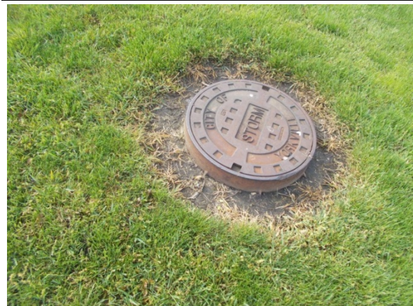
PHOTO #18: STORM SEWER DRAIN
