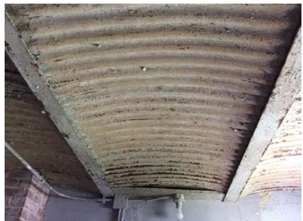
PHOTO #60: CORRUGATED STEEL ARCH FIRST FLOOR FRAMING
