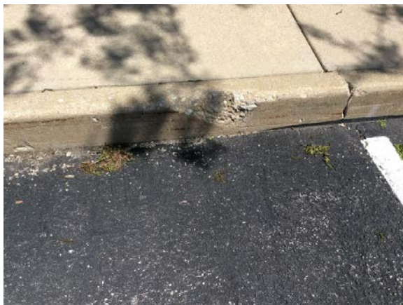
PHOTO #9: CURB, DAMAGED
