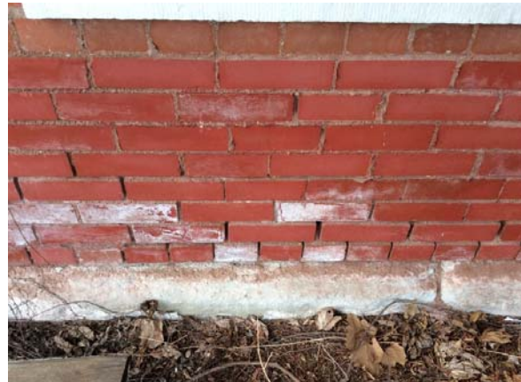
PHOTO #16: EFFLORESCENCE AND MISSING MORTAR
