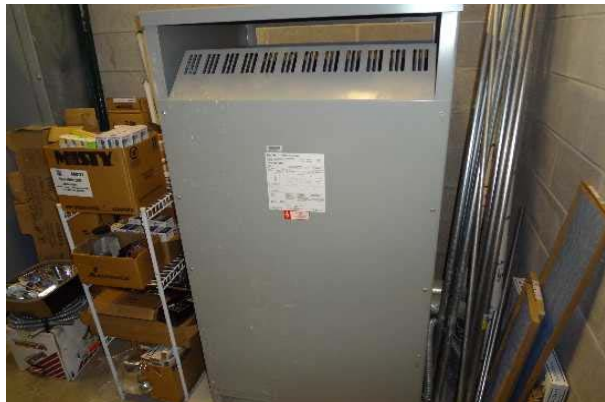
#58: SECONDARY TRANSFORMER, DRY
