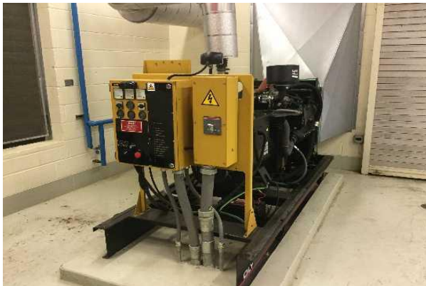
#21: GENERATOR, GAS OR GASOLINE
