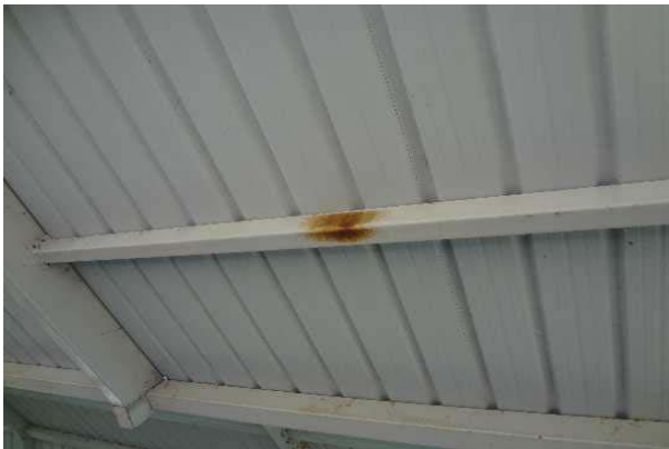
#8: PAINTED SURFACE, SURFACE CORROSION
