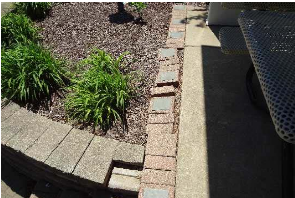
#12: CLAY BRICK/MASONRY PAVERS, MISSING AND DISLODGED BRICKS
