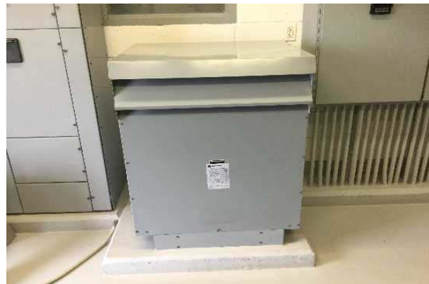
#30: SECONDARY TRANSFORMER, DRY
