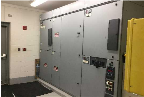
#37: MOTOR CONTROL CENTER W/ MAIN BREAKER
