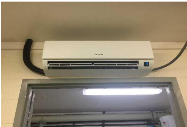
#15: DUCTLESS SPLIT SYSTEM, SINGLE ZONE
