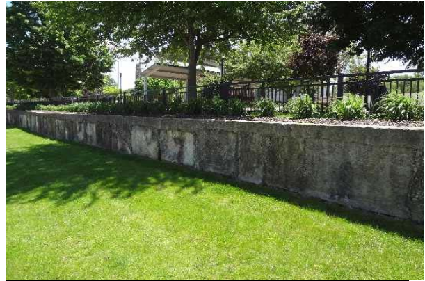
#8: RETAINING WALL, CAST-IN-PLACE CONCRETE
