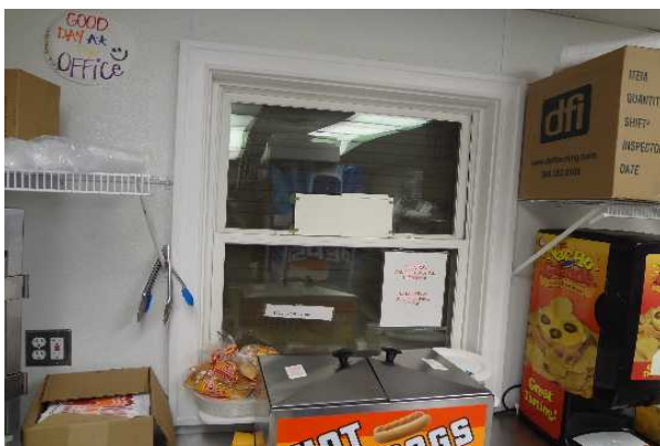
#11: WINDOW, VINYL-CLAD DOUBLE-GLAZED DOUBLE HUNG
