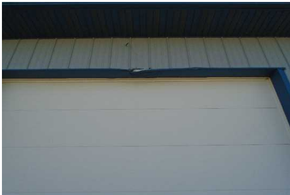
#15: DAMAGE TO OVERHEAD DOOR NO. 5.
