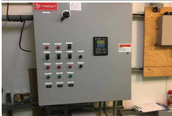
#11: BUILDING AUTOMATION SYSTEM (HVAC CONTROLS)
