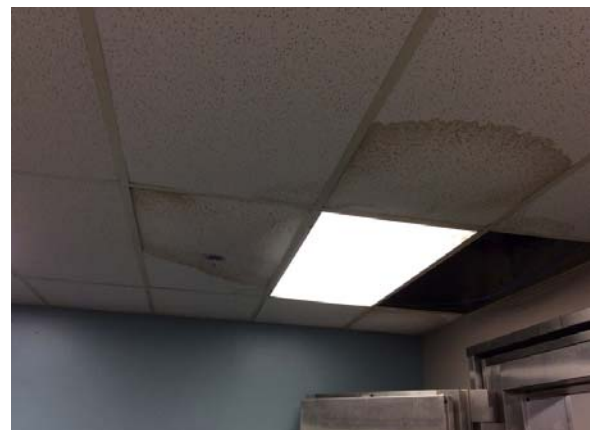
PHOTO #54: WATER DAMAGED CEILING TILE
