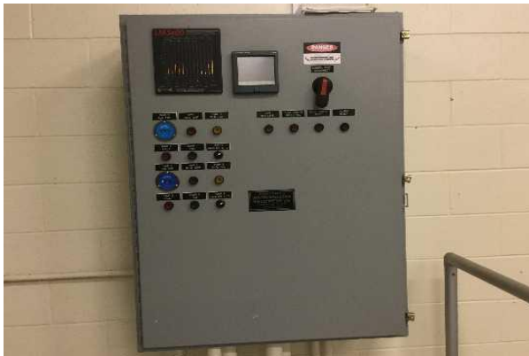
#27: STORM WATER LIFT STATION CONTROLLER
