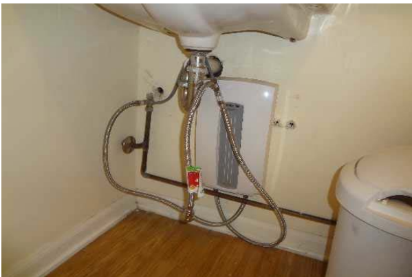
#5: ADA, MISSING LAVATORY PIPE WRAPS
