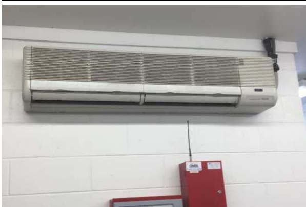
#17: DUCTLESS SPLIT SYSTEM, SINGLE ZONE
