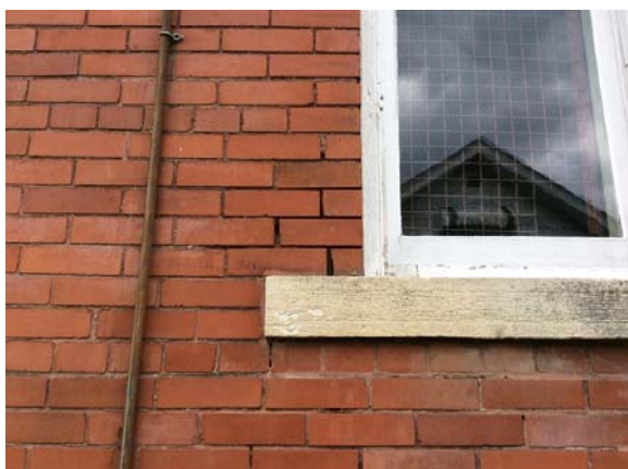
PHOTO #11: MISSING MORTAR
