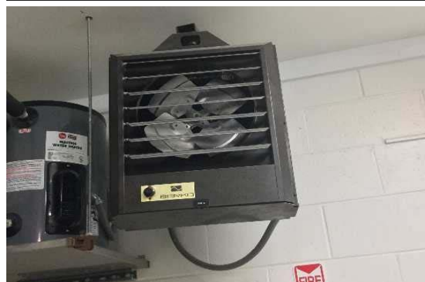
#18: UNIT HEATER, ELECTRIC
