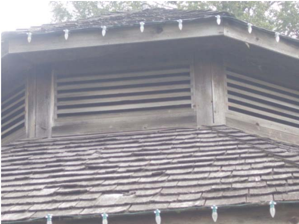
PHOTO #16: CEDAR ROOF SHINGLES
