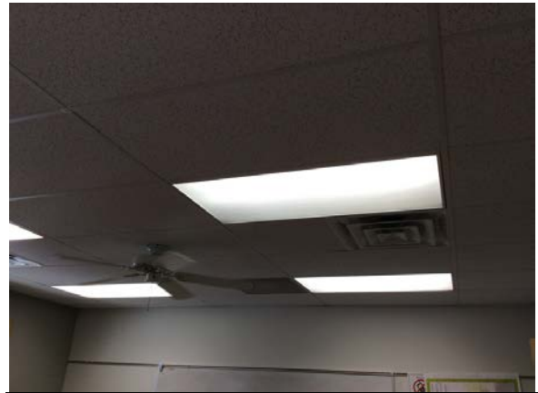
PHOTO #56: ACOUSTICAL TILE CEILING
