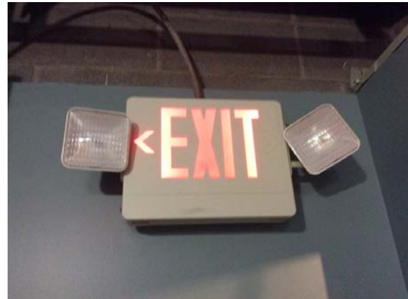
PHOTO #50: EXIT SIGN AND EMERGENCY LIGHT FIXTURE
