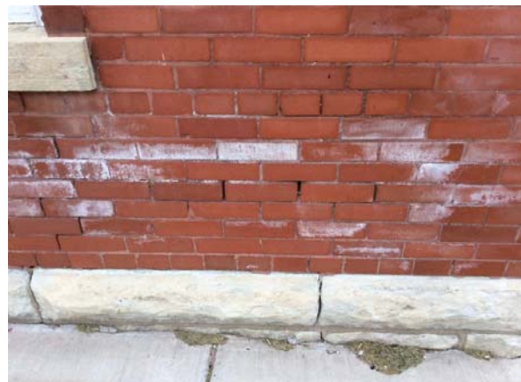
PHOTO #10: EFFLORESCENCE AND DETERIORATED MORTAR
