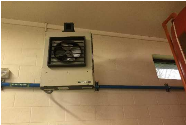
#15: UNIT HEATER, ELECTRIC
