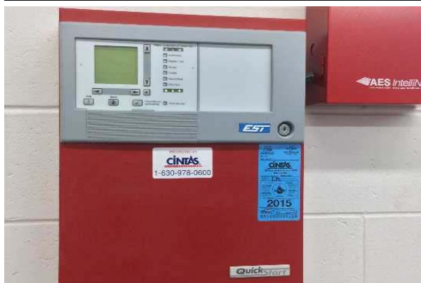
#35: FIRE ALARM CONTROL PANEL, ADDRESSABLE
