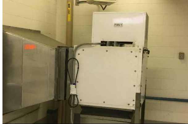
#14: EXHAUST FAN, CENTRIFUGAL
