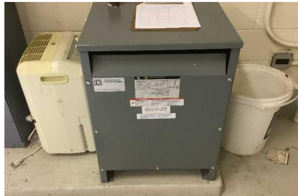
#28: SECONDARY TRANSFORMER
