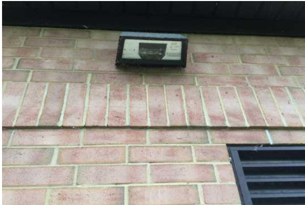
#25: HIGH PRESSURE SODIUM LIGHTING FIXTURE
