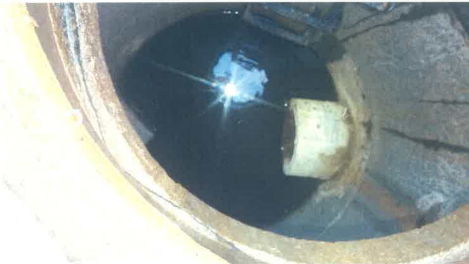
Restrictor Structure 292 with no restrictor on outlet side.
