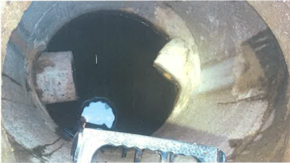
Restrictor Structure 292 with 4" restrictor on inlet side.
