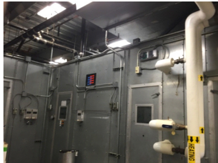
VAV Air Handling Unit
