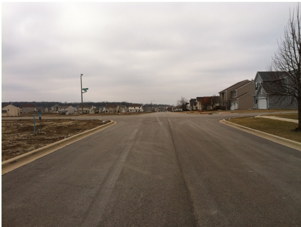
Westbound Approach, Looking West
