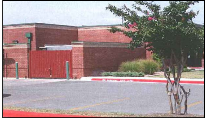
Screen dumpsters with walls and materials that match the architecture of the primary building
