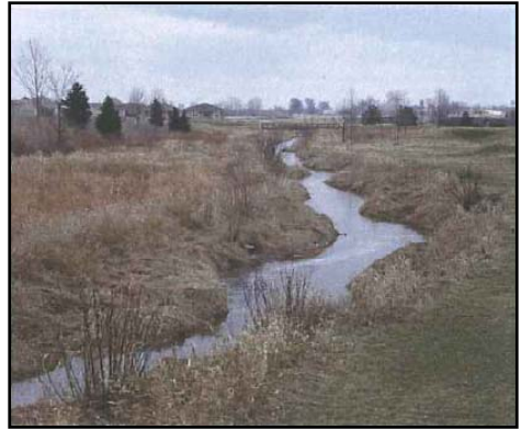
Drainage swale utilizes natural drainage patterns
